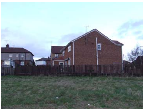
Fig. 5 Housing to the north of the site
