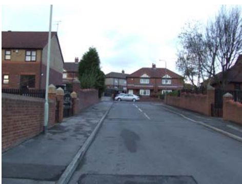
Fig. 7 View north up Alric Drive
