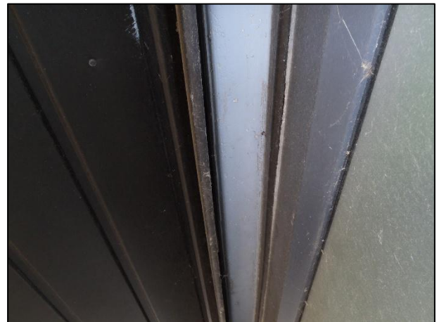
Photograph 6: Gap behind trim over window on south east elevation
