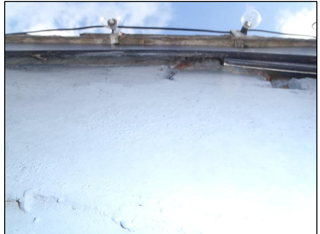
Photograph 12: Gap at south corner of south west elevation
