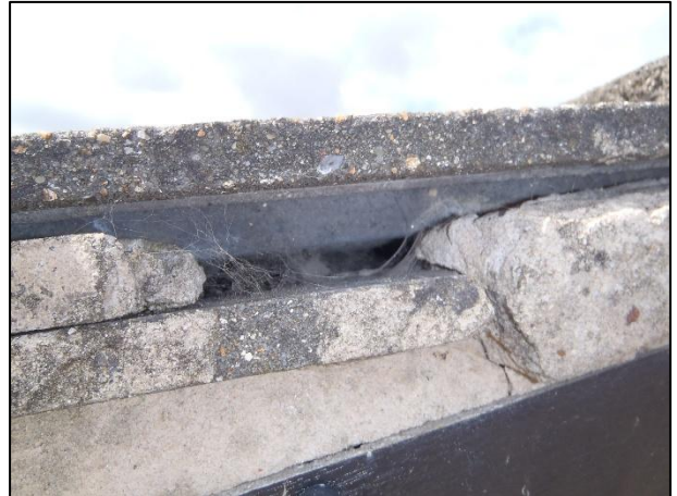
Photograph 10: Gap under trim below gable verge on south west elevation
