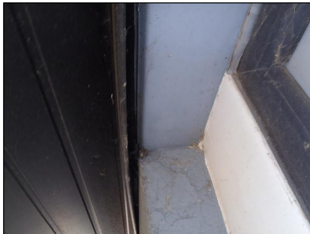
Photograph 5: Gap behind trim at wall top on south east elevation
