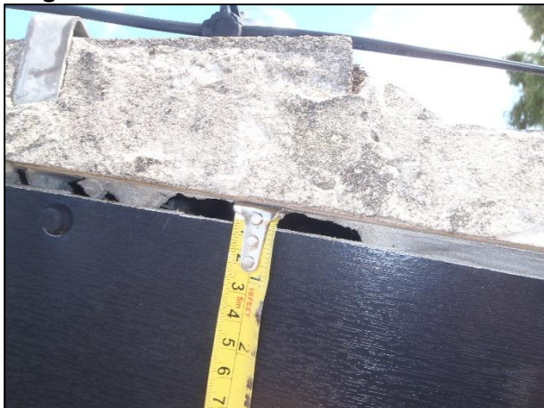
Photograph 11: Gap above trim at gable verge on south west elevation
