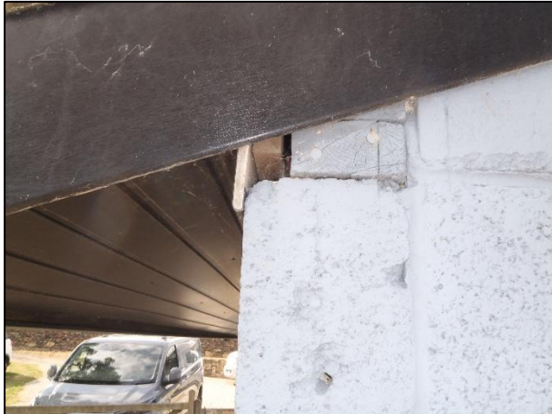
Photograph 9: Gap under trim below gable verge on north east elevation
