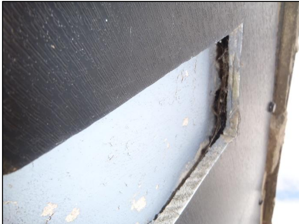
Photograph 11: Gap above trim at gable verge on south west elevation
