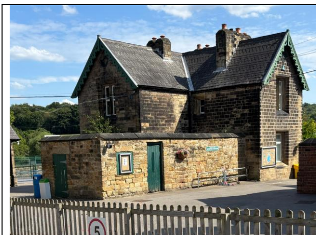
Photo 6 – External face of retained stone boundary wall showing differing in material
