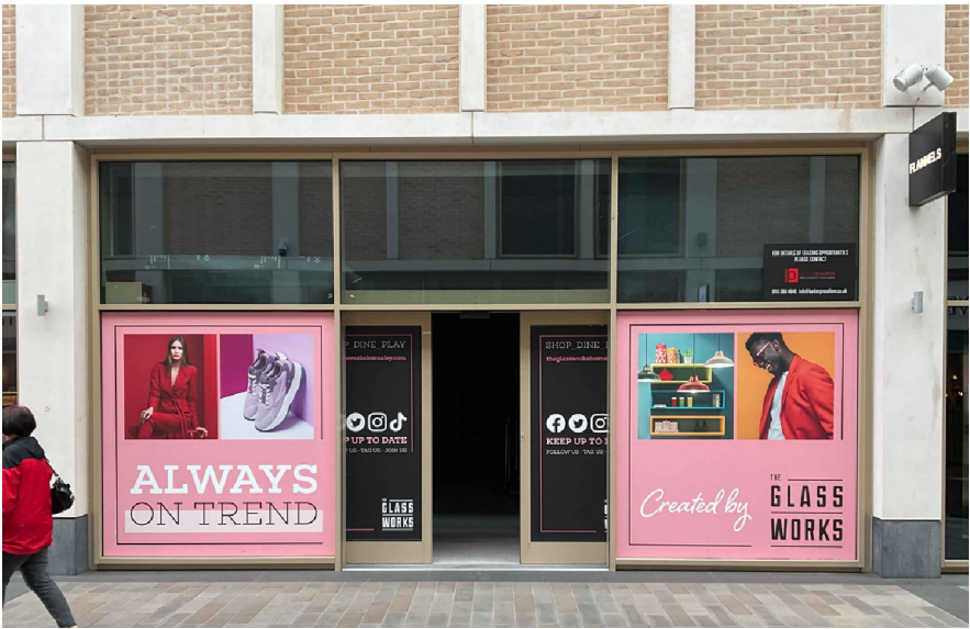
GENERAL PHOTO OF FRONT FACING ELEVATION
