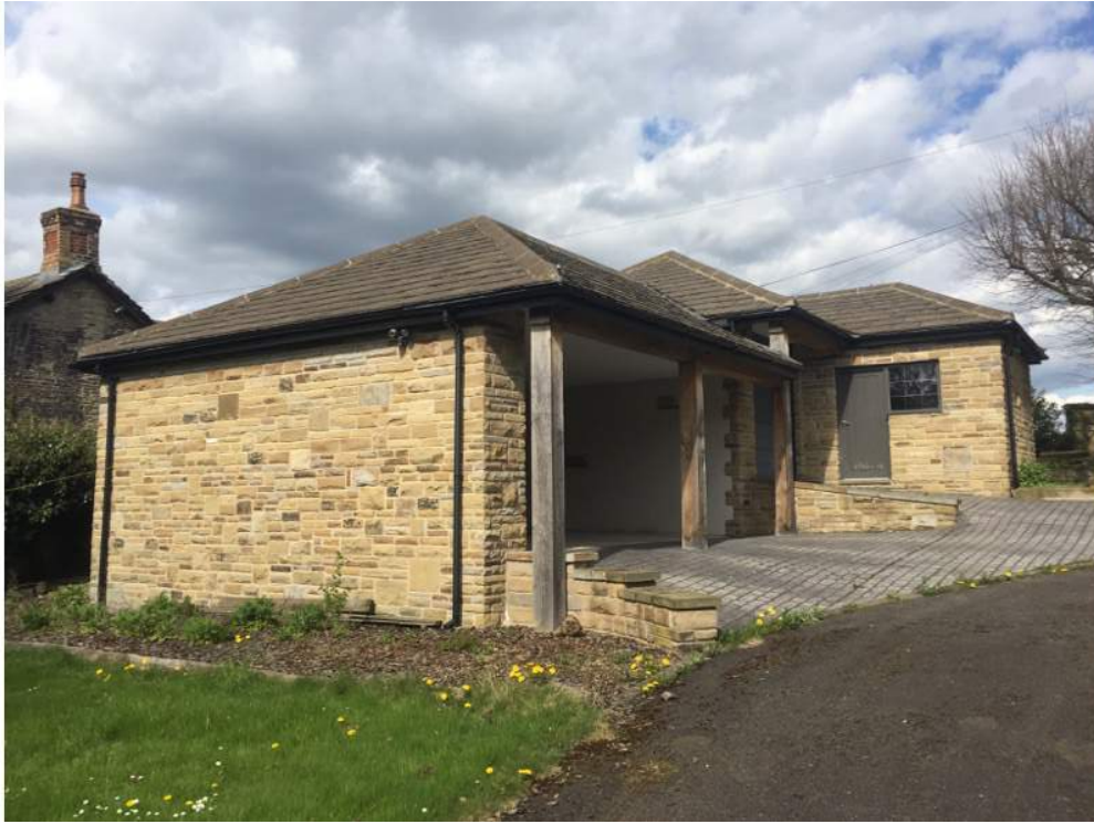
Fig. 03 – Photo of Existing Garage from the south west
