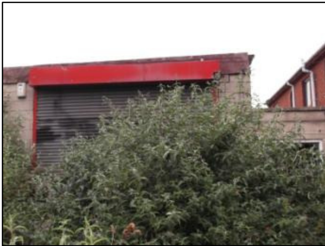
Photograph 7: External of B4
