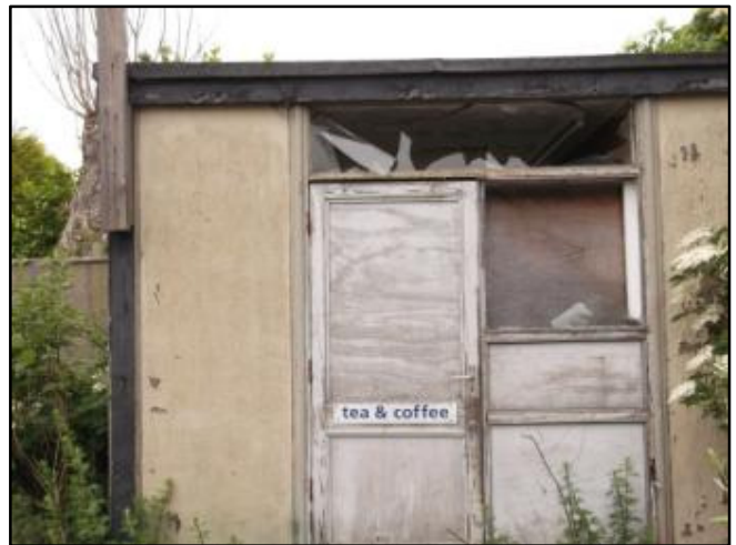
Photograph 10: External of B6
