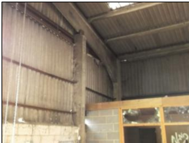
Photograph 2: Internal of B1
