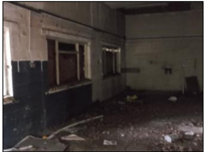
Photograph 8: Internal of B4
