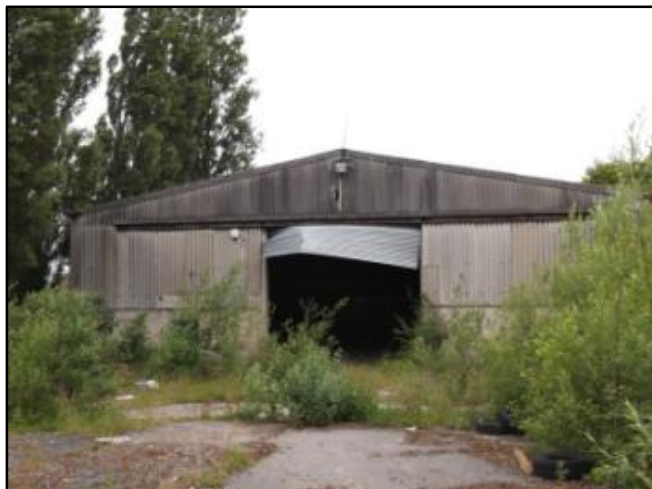
Photograph 1: External of B1
