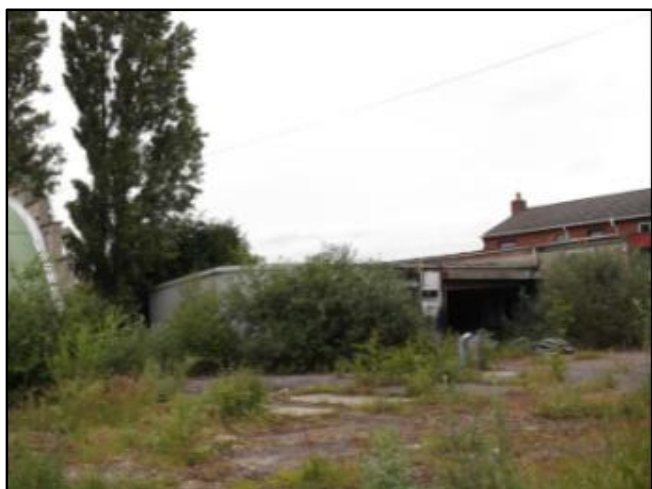
Photograph 5: External of B3
