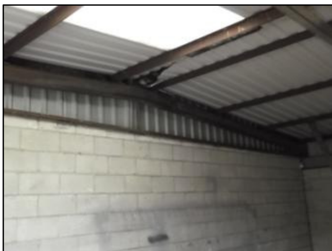
Photograph 6: Internal of B3
