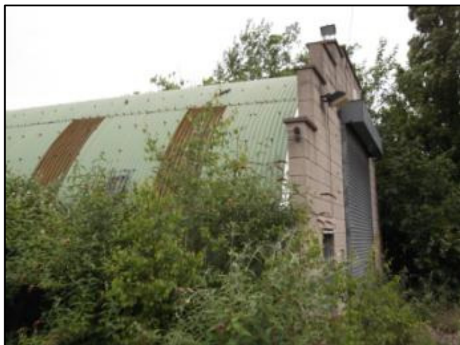
Photograph 3: External of B2
