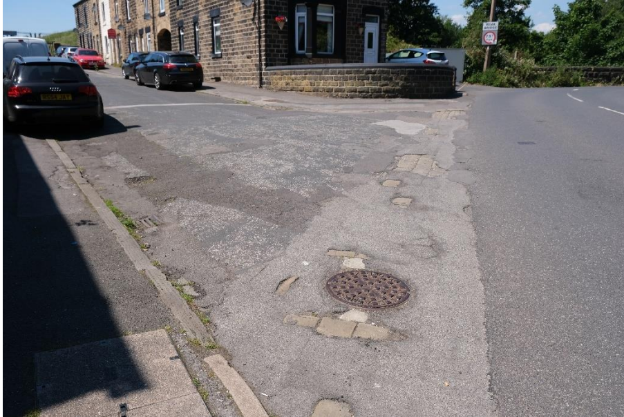
Photograph 6: Existing road surface on Hopewell Street and Hoyle Mill Road junction.
