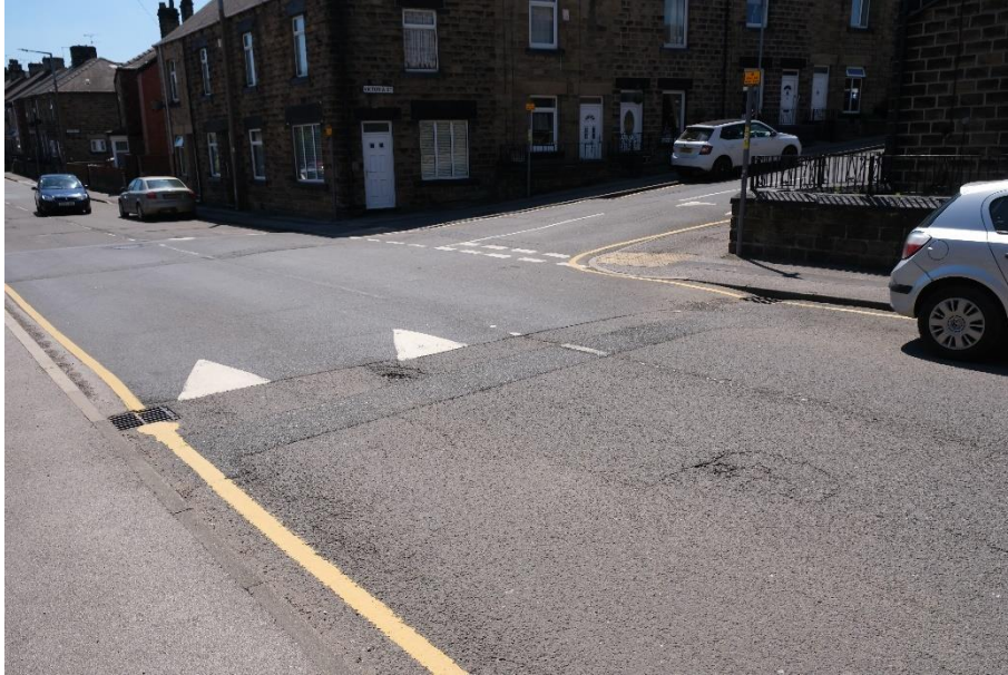
Photograph 12: Existing road surface on Hoyle Mill Road junction with Victoria Street.
