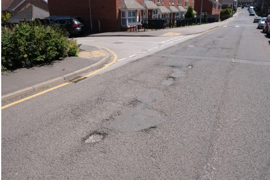
Photograph 10: Existing road surface on Hoyle Mill Road junction with Sheepcote Walk.
