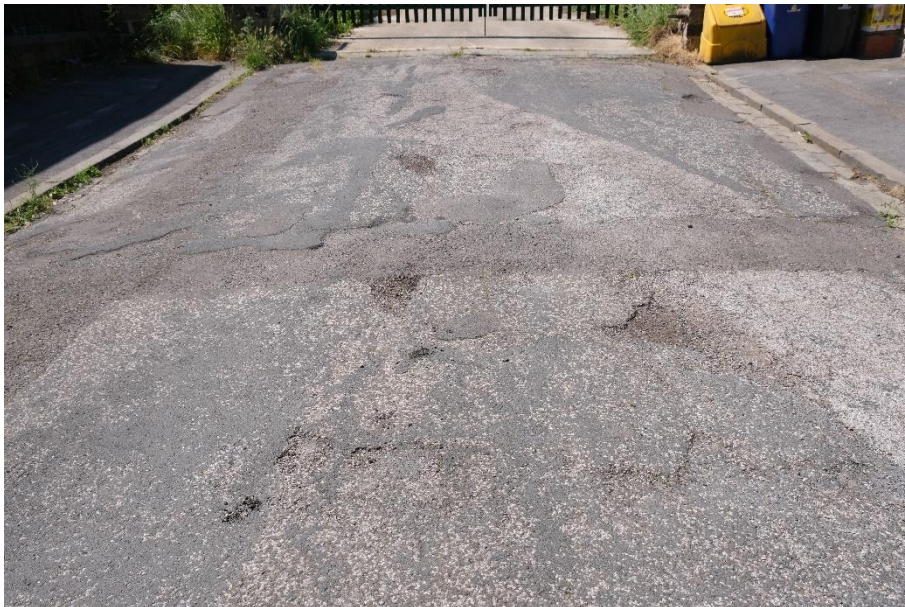
Photograph 3: Existing road surface on Hopewell Street prior to site access.
