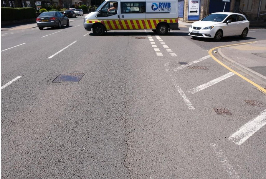
Photograph 18: Existing road surface on A635 Doncaster Road just east of junction with Hoyle Mill Road.
