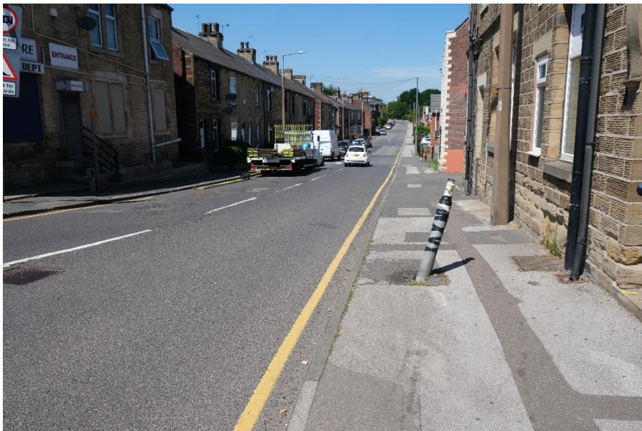
Photograph 19: Existing footway and signpost on Hoyle Mill Road just north of junction with A635 Doncaster Road.
