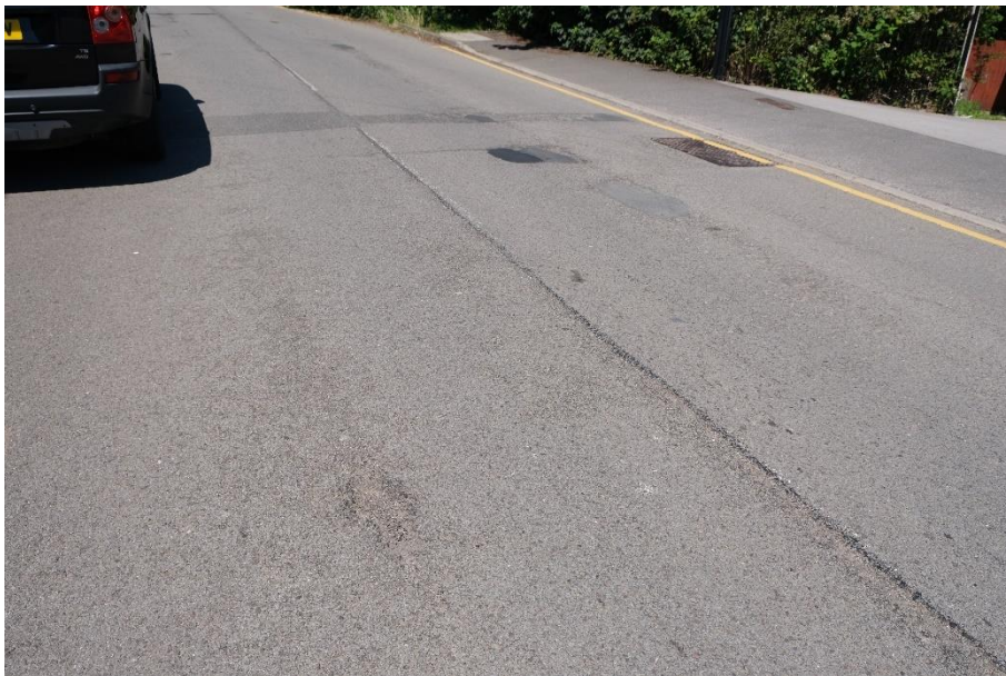
Photograph 9: Existing road surface on Hoyle Mill Road.
