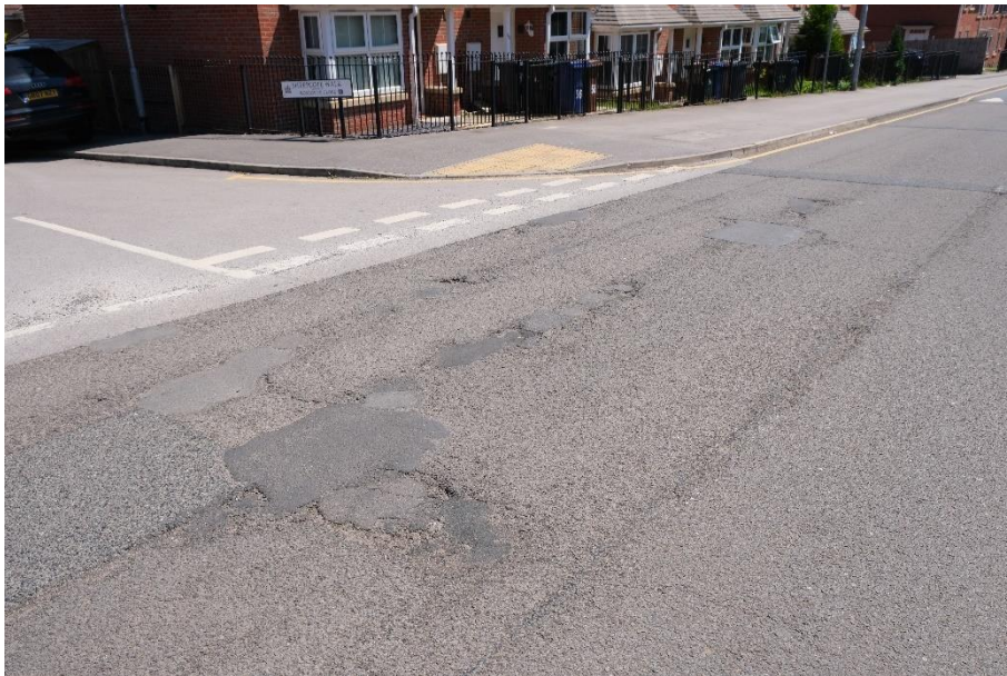
Photograph 11: Existing road surface on Hoyle Mill Road junction with Sheepcote Walk.
