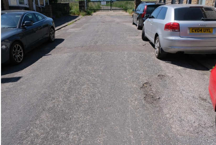
Photograph 4: Existing road surface on Hopewell Street.
