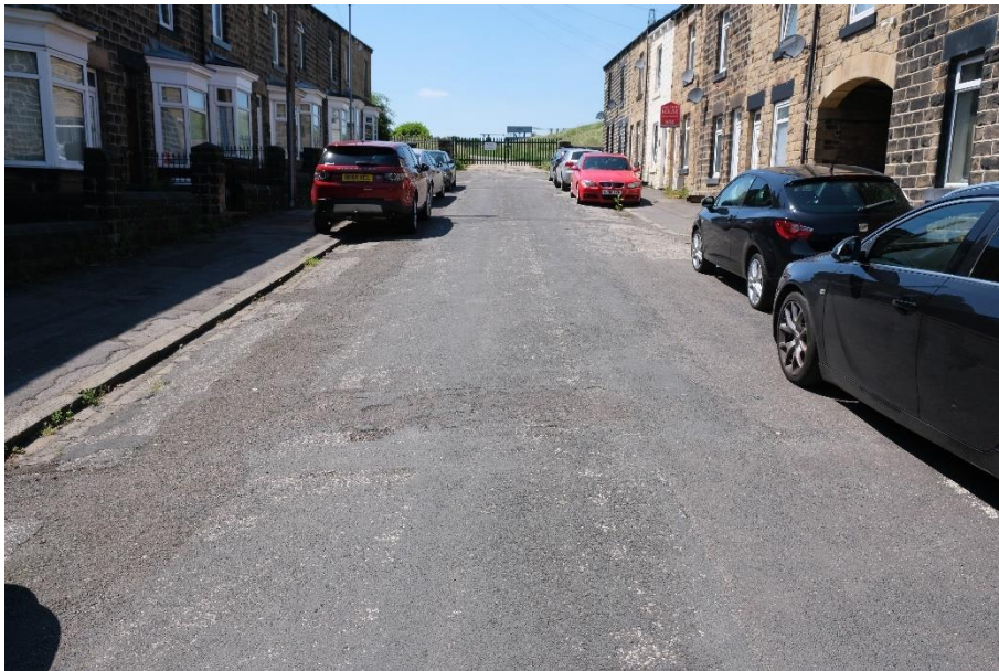
Photograph 5: Existing road surface on Hopewell Street.
