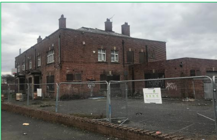
The north and west elevation of the building
