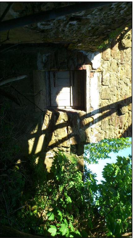
PICTURE P SHOWING MISSING SECTION OF EXTERNAL WALL IN AREA OF FIRST FLOOR LOADING DOORS AND ACCESS STAIR
