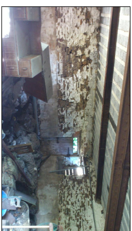
PICTURE I INTERNAL VIEW SHOWING FIRST FLOOR CONSTRUCTION
