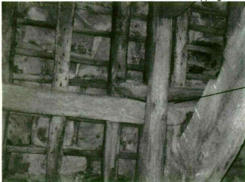
Plate 6 Internal view of the roof to illustrate overlapping roof timbers
