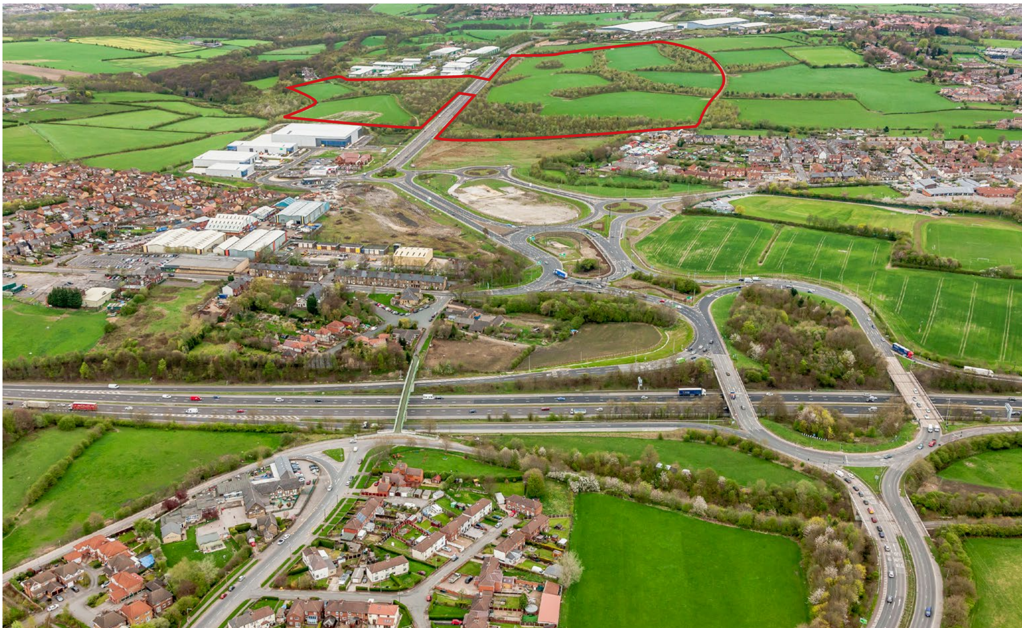
Aerial photograph looking East over Junction 36 of the M1
