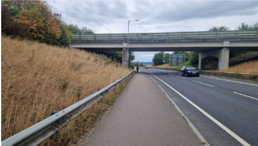
IMG-2: Cudworth Parkway (A628) Adjacent To NM1 (Site Top Of Left Bank)
