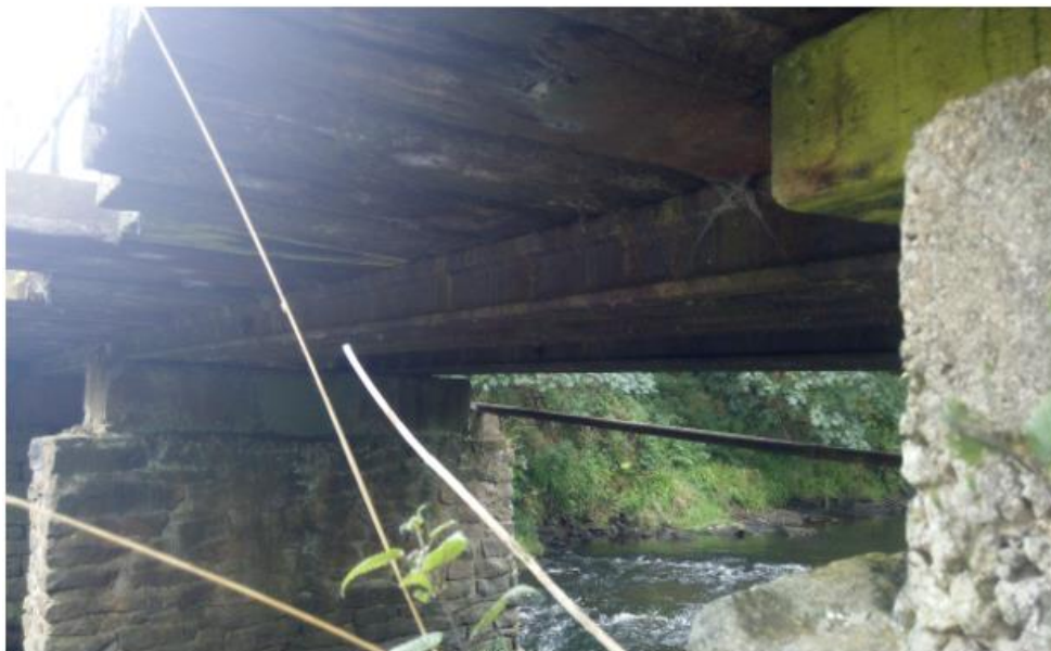
Above: Fig 1.5.2 View on underside
