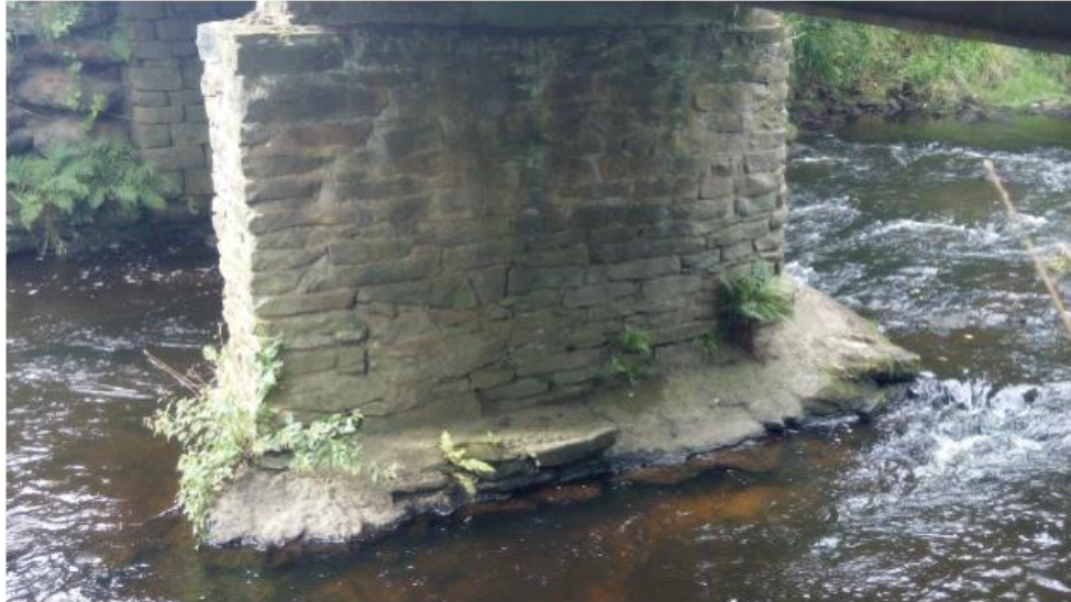
Above: Fig 1.5.3 View on Central Pier
