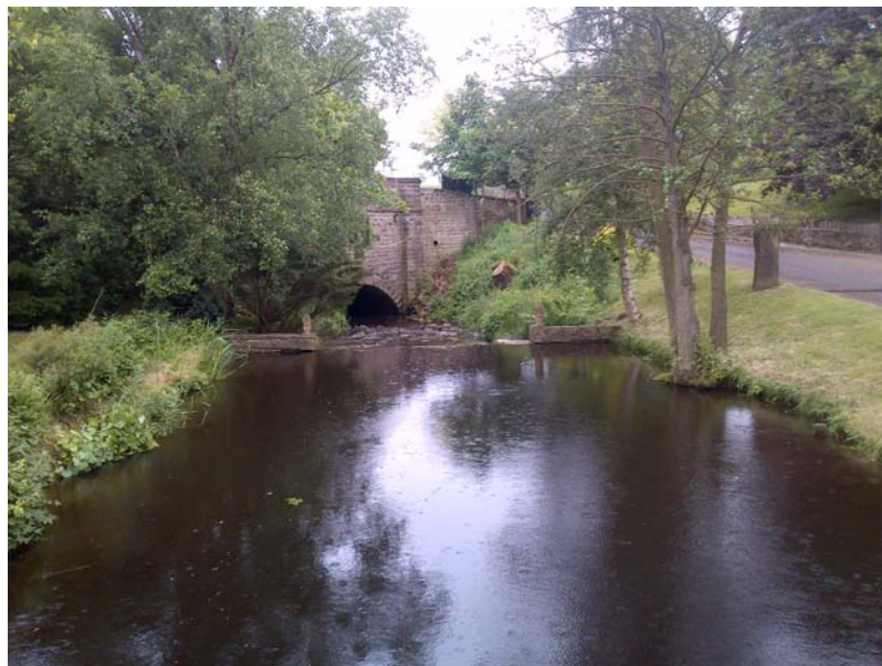
Figure 4.1: View downstream towards Huddersfield Road Bridge.
