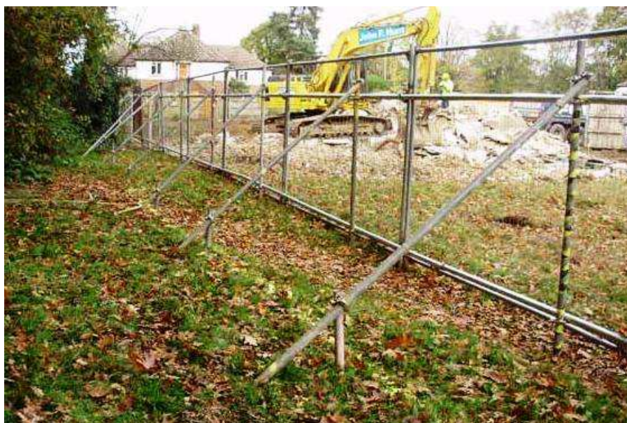
Figure 2: 'Photo of Fencing to BS 5837: 2012'.
