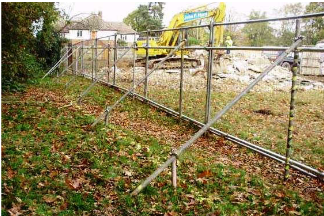
Figure 2: Photo of Fencing to BS 5837: 2012
