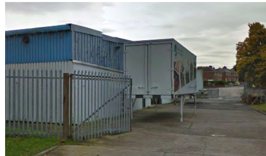
Neighbouring unit off Tinsley Road
