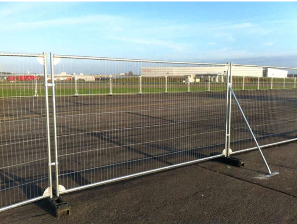
Inset 2: Photo of tree protection fencing
