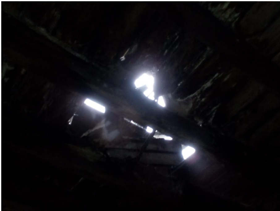
Image 8: B3 interior - showing gaps in roof
