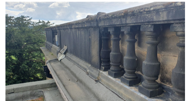
3.11 Sandstone parapet and balustrading
