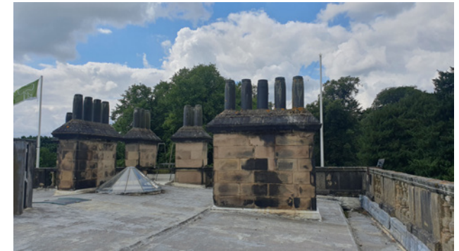
3.9 View across the central block roof
