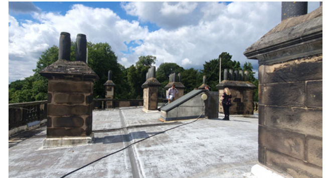
3.16 General state of weathering of the asphalt roof covering
