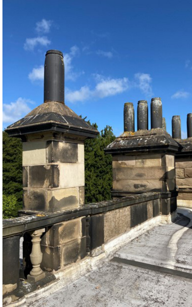
3.22 Past stonework repairs to the chimney stacks.
