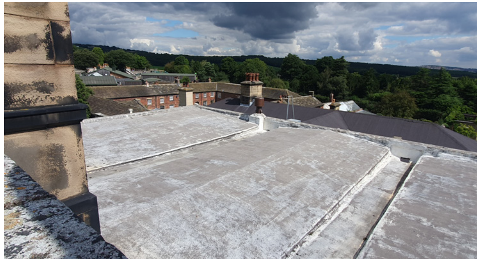
3.15 Eastern flanking wing roof
