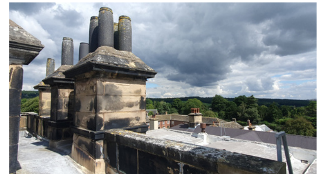
3.10 Chimneys on the central block roof
