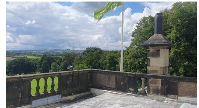
3.6 Stone parapet and balustrading, and views looking south
