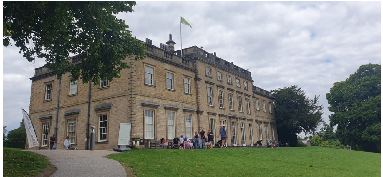
3.4 South garden elevation of Cannon Hall
