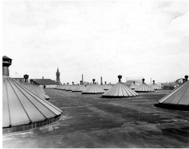
3.14 Temple Works roofscape in the late 20 th century, showing the replacement conical skylights that survive today
