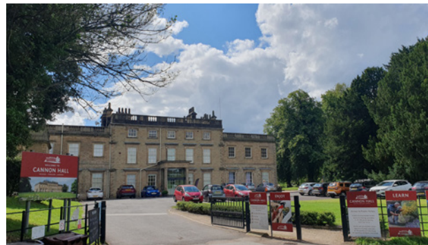
3.5 North elevation of Cannon Hall
