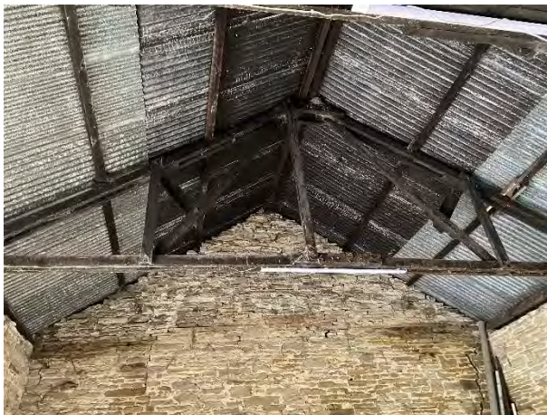
Figure 34: Barn Timber Roof Truss
