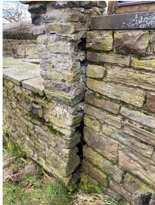
Figure 9: Interface Between the Patio and Conservatory Retaining Wall
