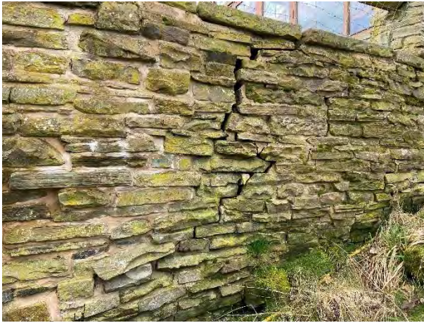
Figure 8: Patio Retaining Wall
