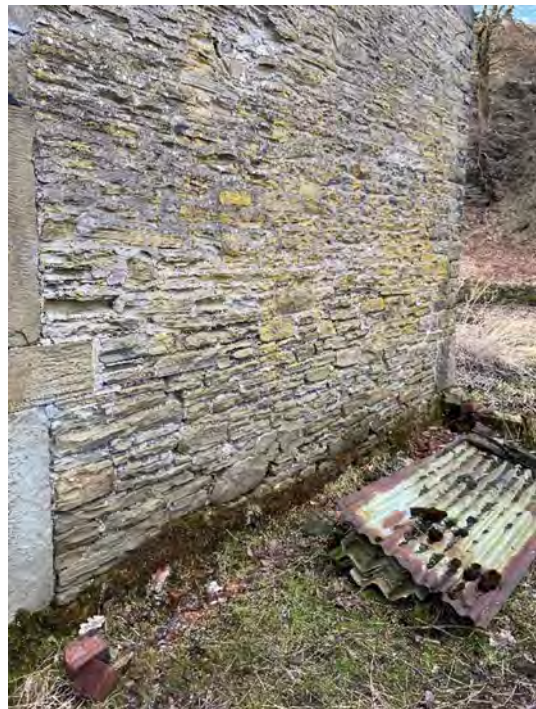
Figure 35: Barn Rear Wall 1
