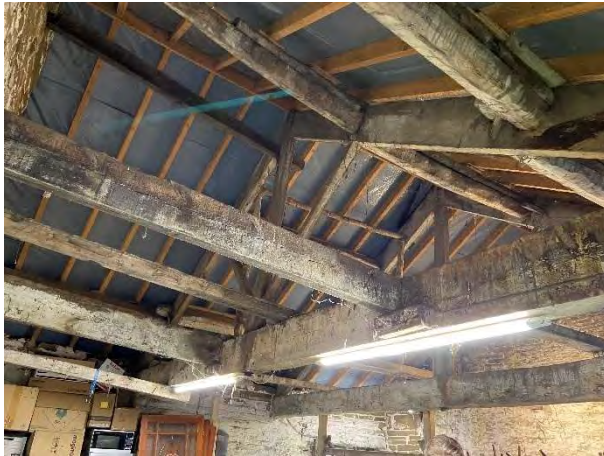
Figure 16: Workshop Roof Structure
