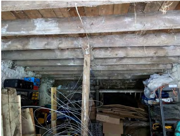
Figure 27: Propped Timber Floor
