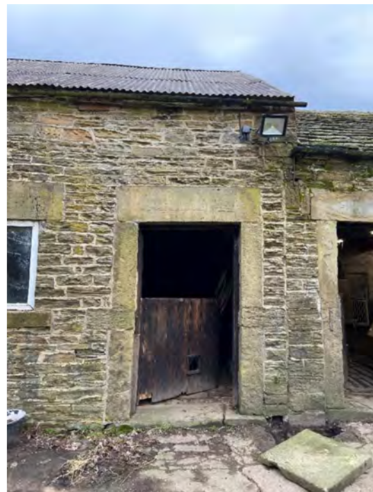
Figure 22: Barn Personnel Door Entrance
