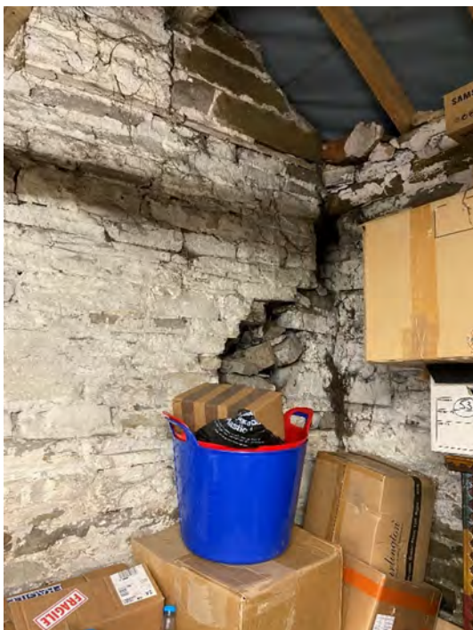
Figure 18: Workshop Internal Wall
