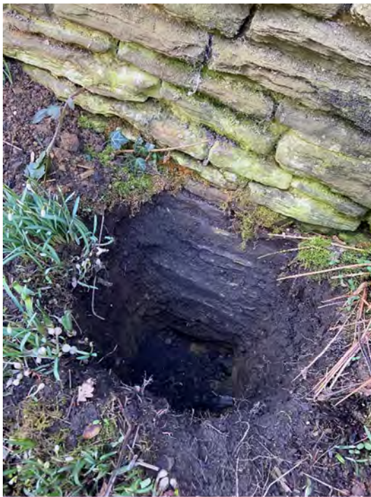
Figure 40: Trial Pit 6 Arisings
