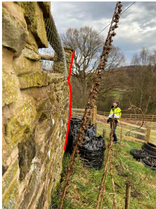
Figure 7: Patio Retaining Wall (Wall Profile Highlighted)
