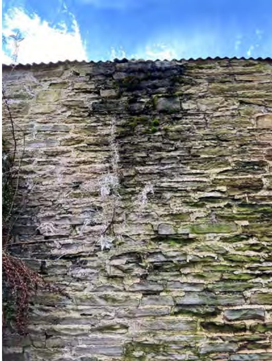
Figure 36: Barn Rear Wall 2
