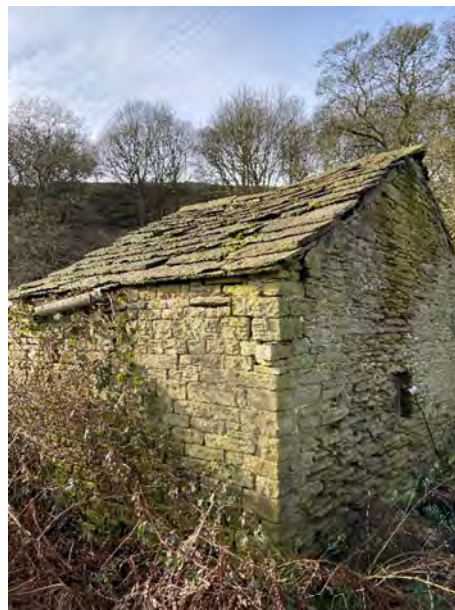
Figure 41: Slaughterhouse North and East Elevations
