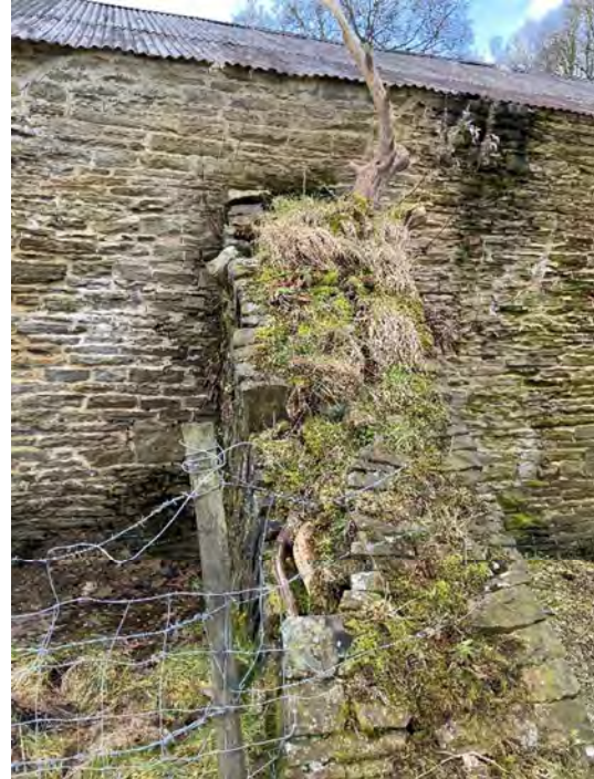
Figure 37: Barn Rear Buttress
