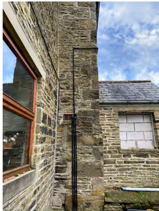
Figure 11: Farmhouse Step in Rear Elevation
