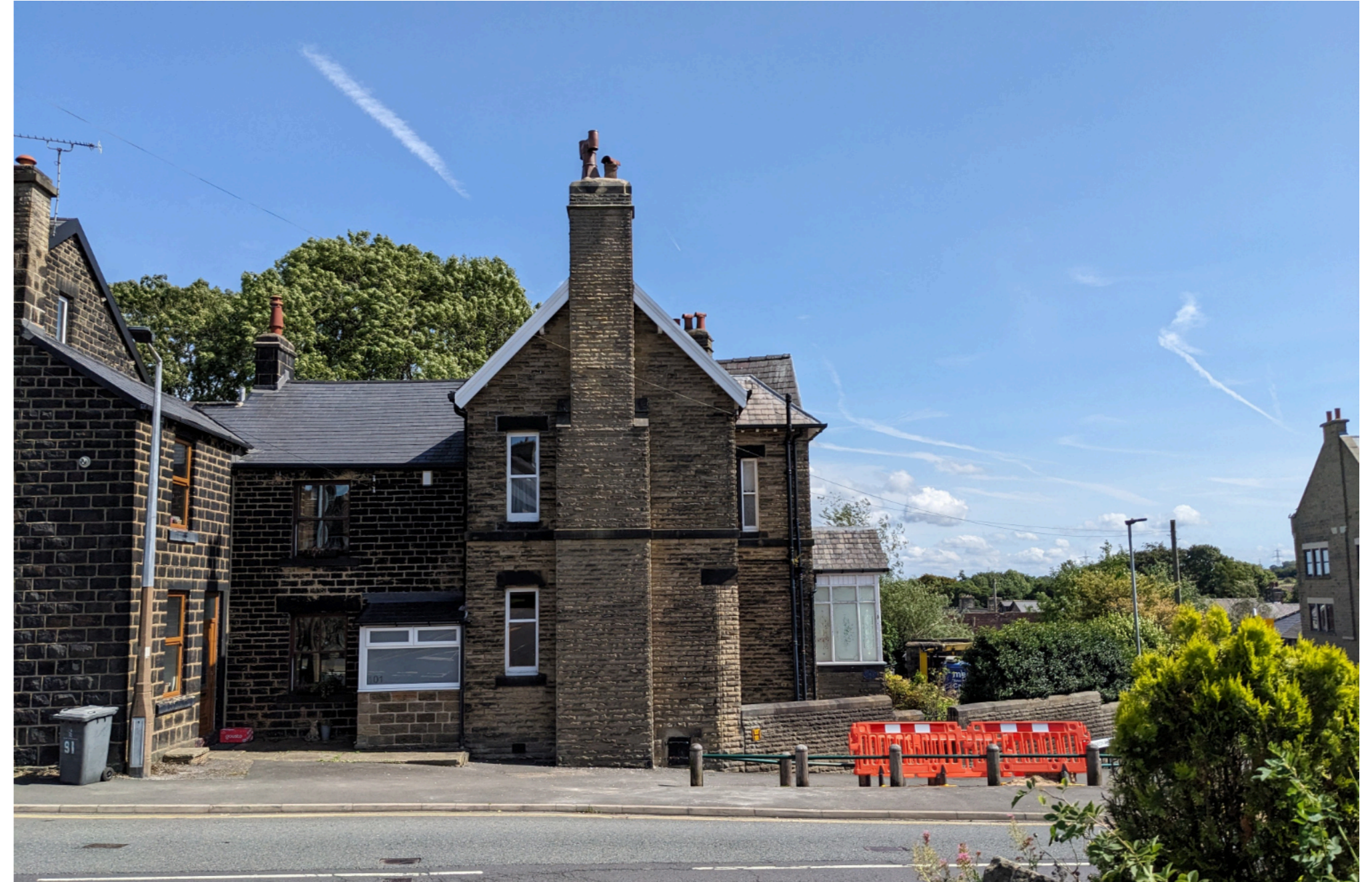
2306 - 103 High Street, Penistone Side (West) elevation viewed from High Street
