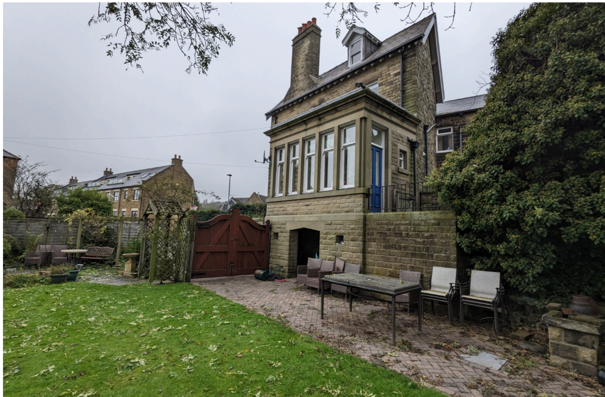
2306 - 103 High Street, Penistone Side (East) elevation viewed from private garden
