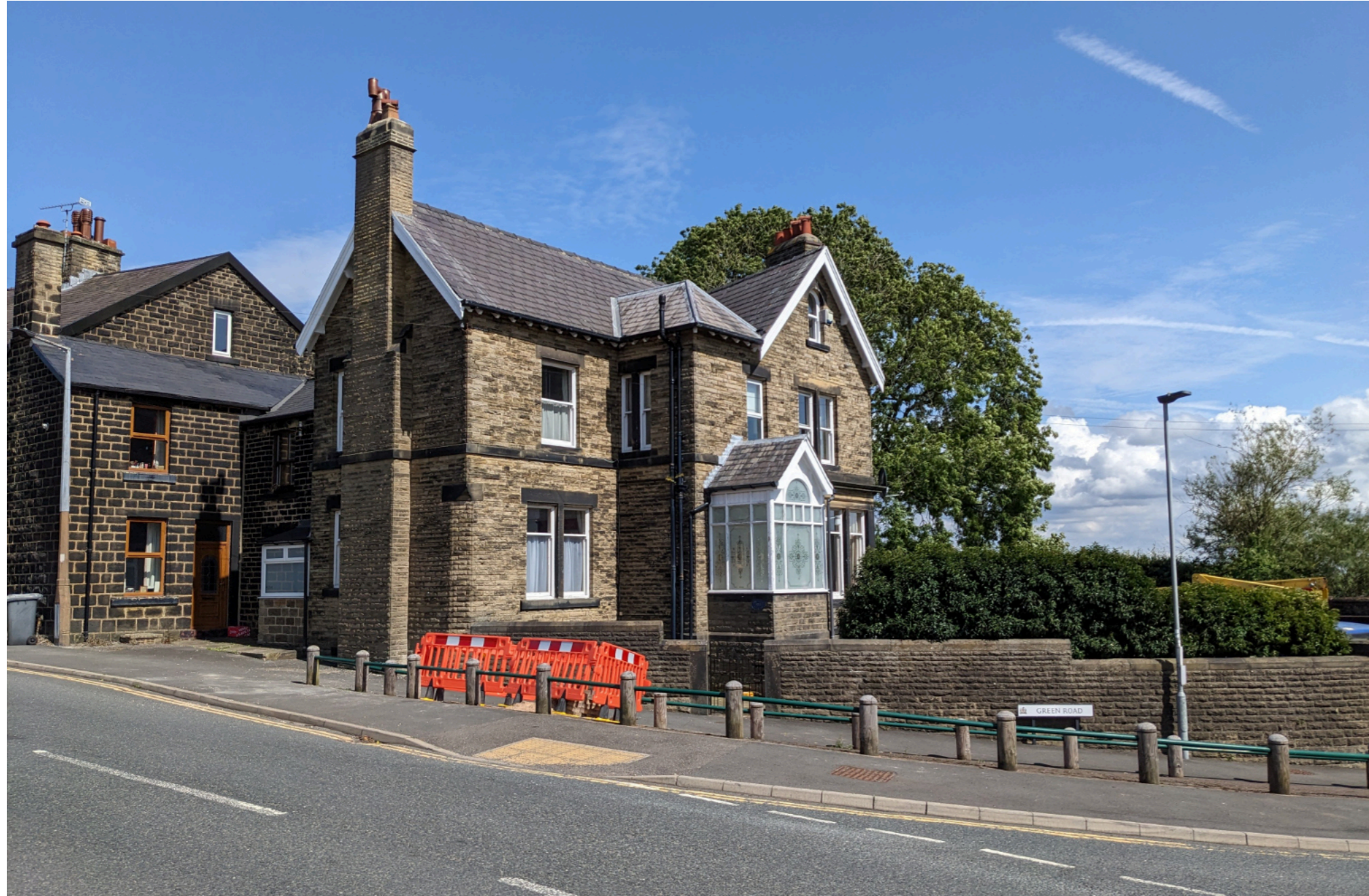
2306 - 103 High Street, Penistone Front (South-west) elevation viewed from High Street
