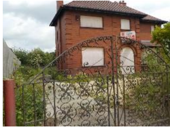
Fig 2: Photograph showing the entrance to the site
