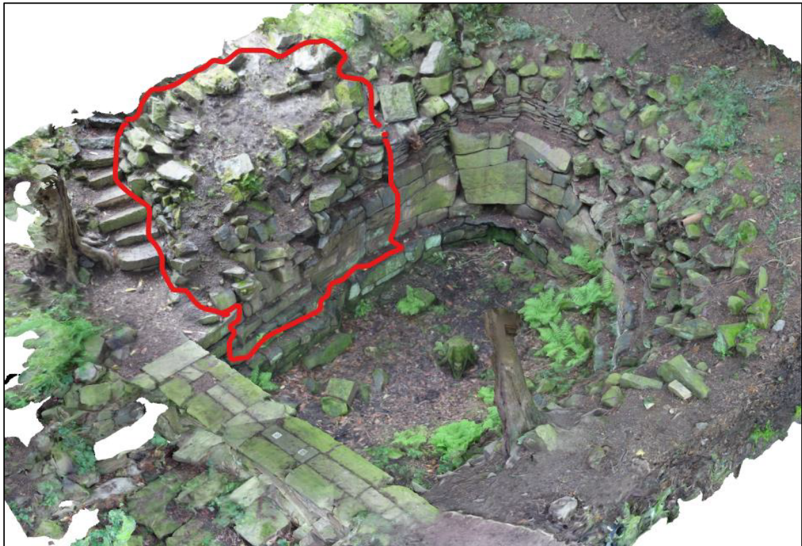
Figure 2: Birdseye view of the Plunge Pool, looking north-west, showing the area to be rebuilt
