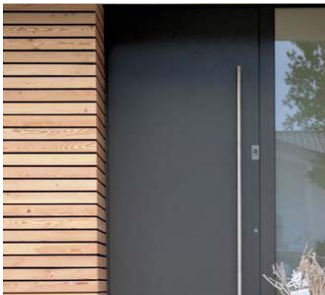
Aluminium doors and windows, with timber external stores to each property
