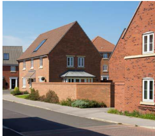
Walls to site frontage in same brick type as dwellings
