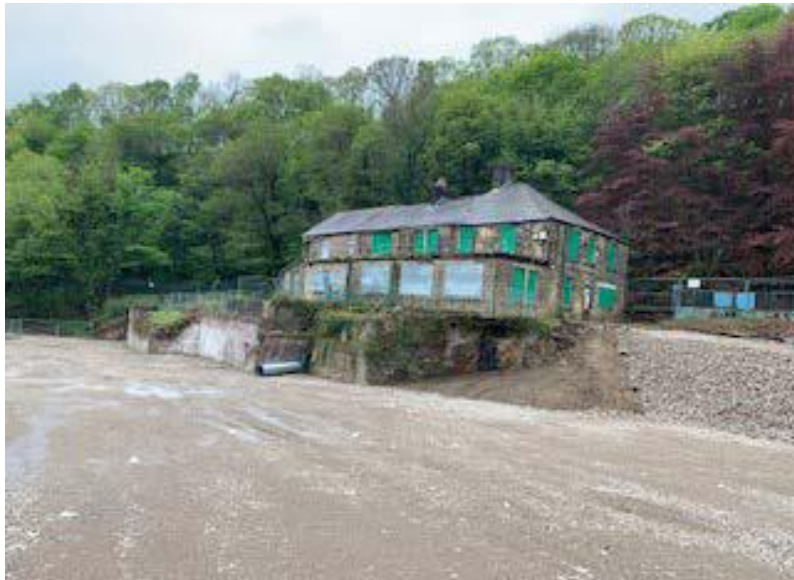
Existing building to be retained & refurbished into 4 new apartments and 1 x 3 bedroom cottage.
