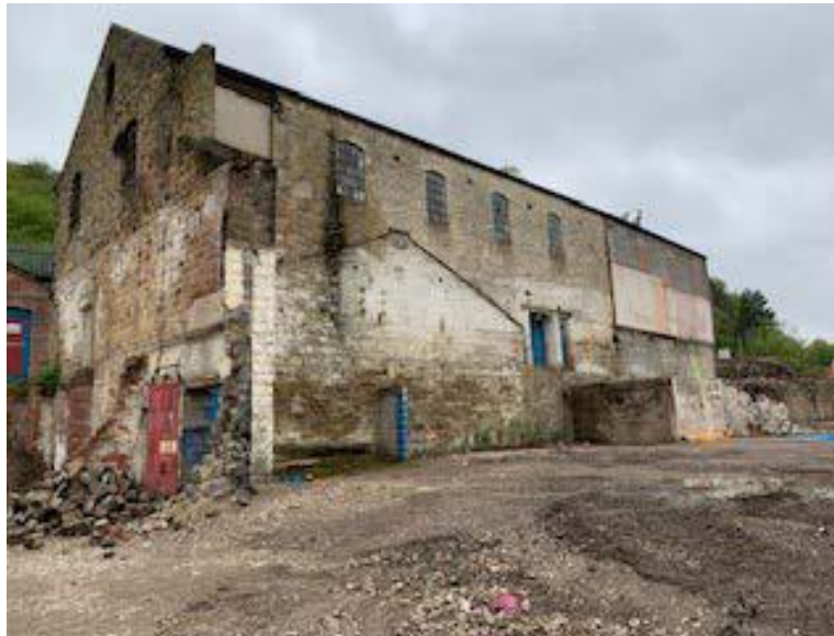
View of existing mill to be refurbished into 8 new apartments.
