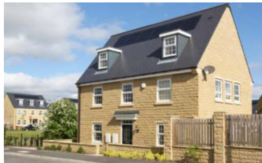
Artstone piers and panel walls to corners
