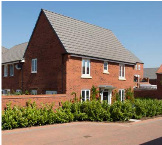
Low level informal landscaping with street trees to front gardens along main spine road.
