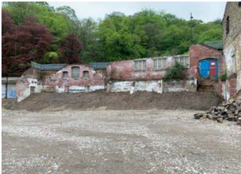
Remains of the demolished buildings to the roadside - to be cleaned and enhanced to provide a sound barrier to new dwellings.
