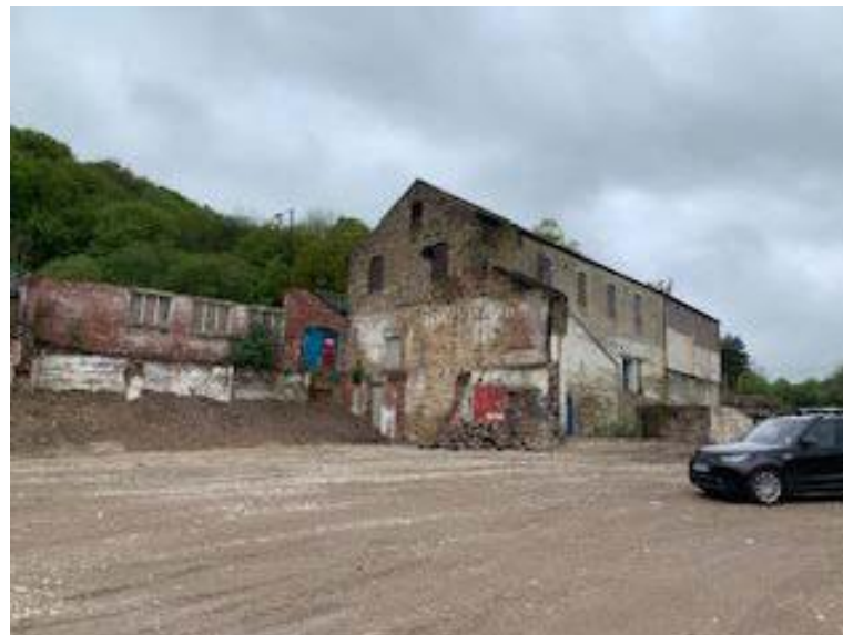
View of existing mill to be refurbished into 8 new apartments.
