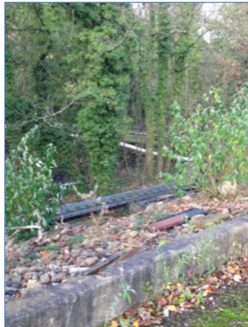
Photograph 6. Rubble and scrub area at TN3, next to the River Don
