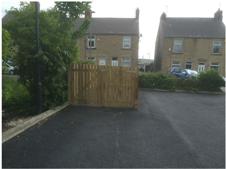
Existing Bin Store
