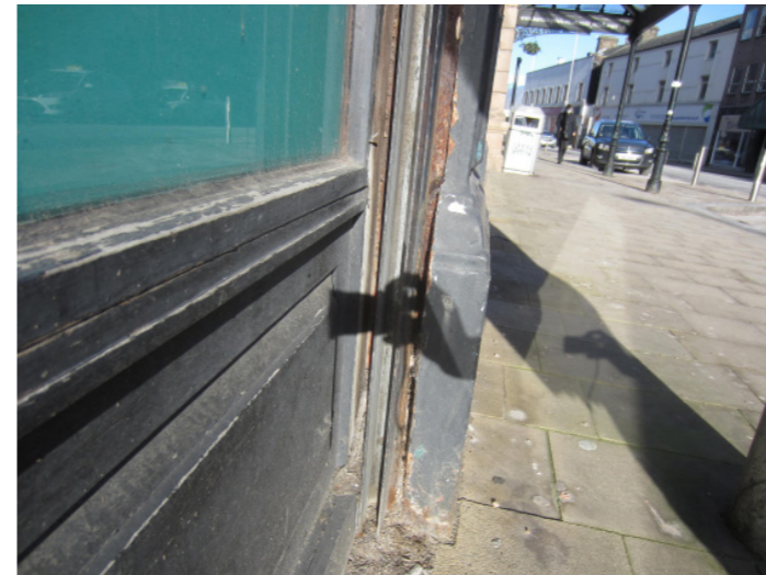
Existing cast iron pilasters
