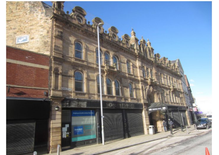
Existing Eldon Street Facade
