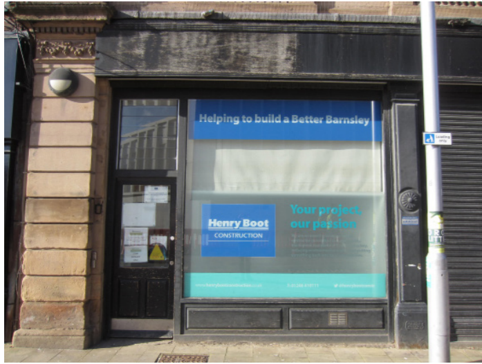
Secondary entrance on Eldon Street facade
