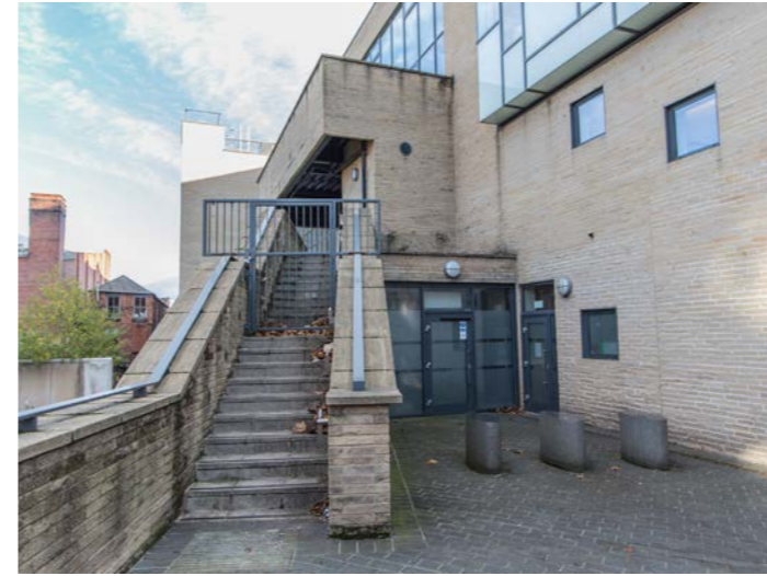
Existing staircase to access the second floor balcony
