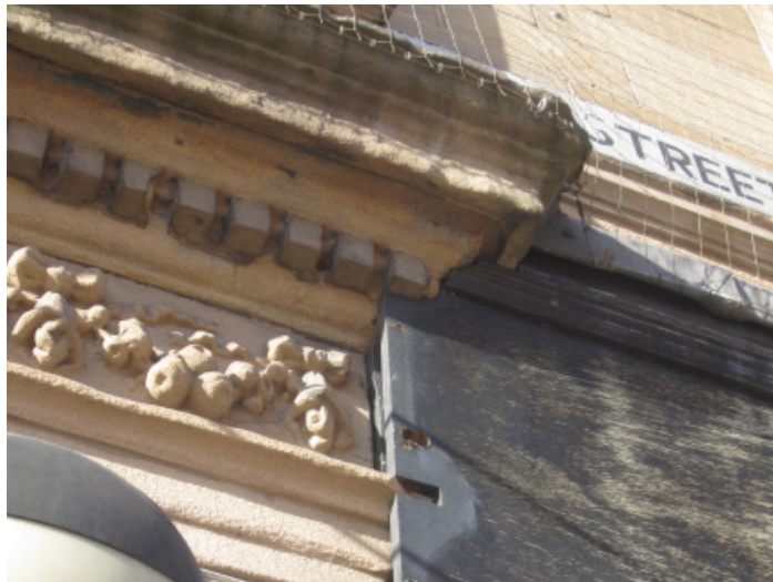
Existing signage and fascia detail
