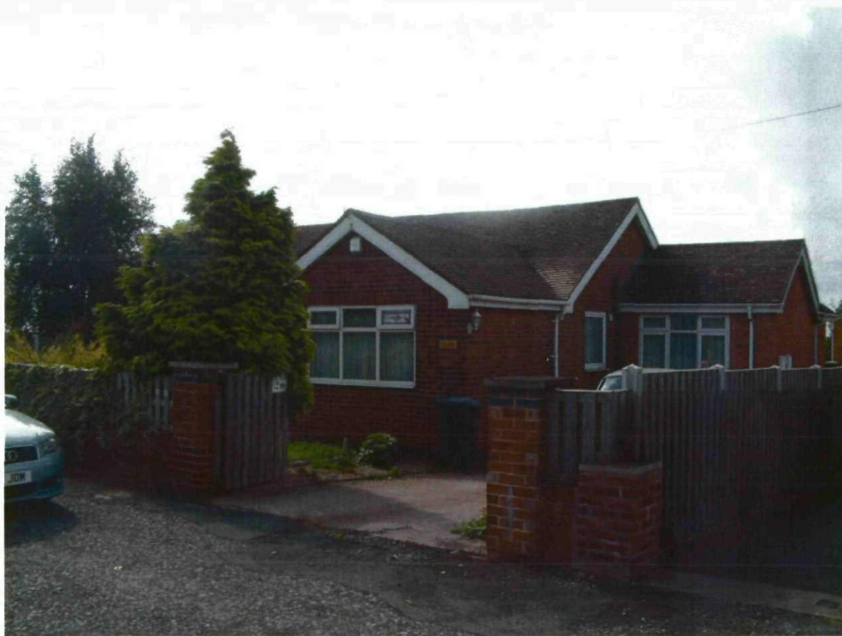
Photograph above shows front of existing property No 569 Doncaster Rd
