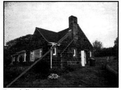
Lead flashing gap.
