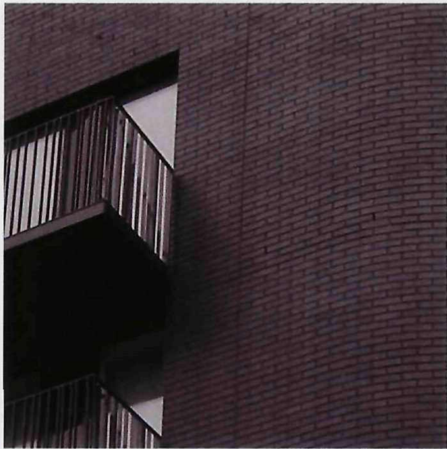
Dark facing brickwork tied back to blockwork system
