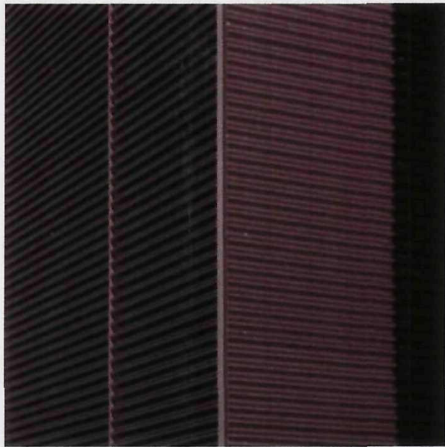
Black sinusoidal metal profiled cladding - illustrating fin joint
