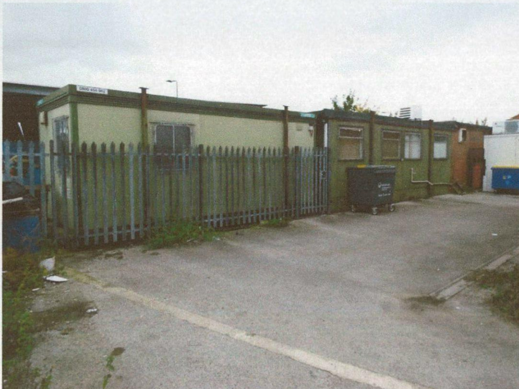
Photograph No.3 - View from rear yard (south eastern boundary)
