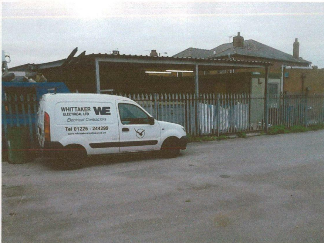
Photograph No.4 - View from adjacent yard (south western boundary)
