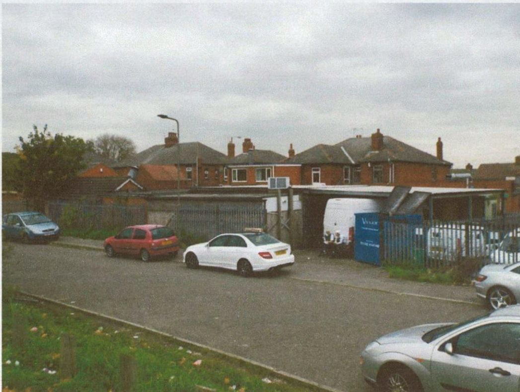
Photograph No.1 - View from the rear Service Road
