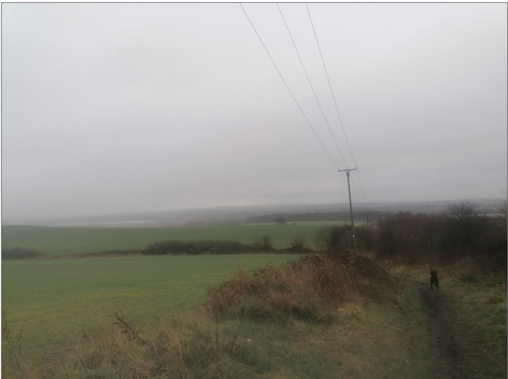
Plate 28: View of Area 4 looking south-west down the tramway from the south-west of Brierley.
