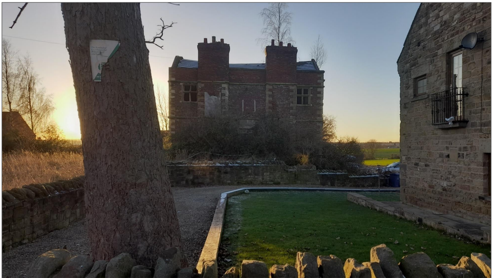
Plate 30: Grimethorpe Hall, looking towards the north-east facing elevation.
