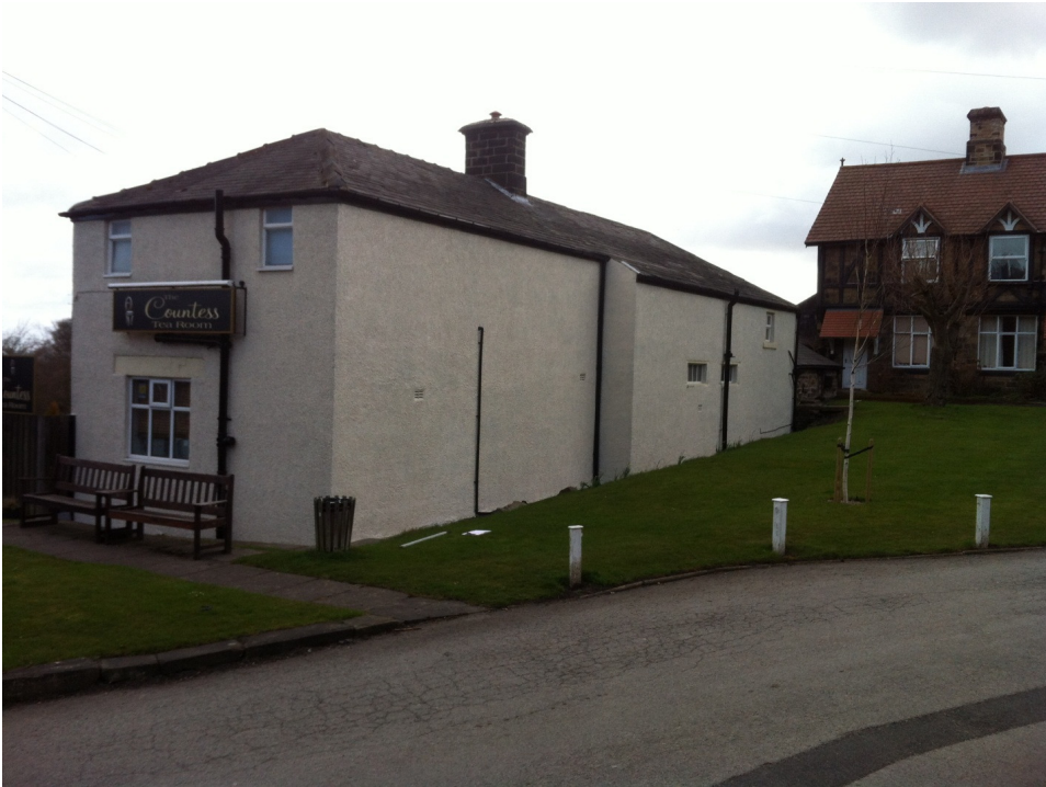
1. South East and South West (rear) elevation viewed from Halifax Road.
