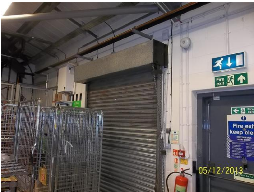
Roller Shutter No.7 Internal (External View)
