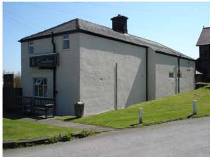
Fig 1 South West (rear) and North West (end) elevations
