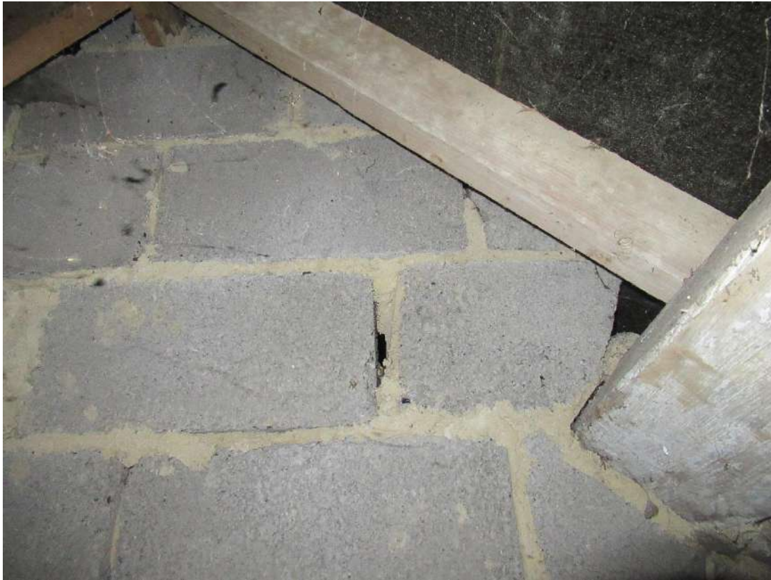
Photograph 15: Interior view of Building 2, with cavities in the breezeblock.
