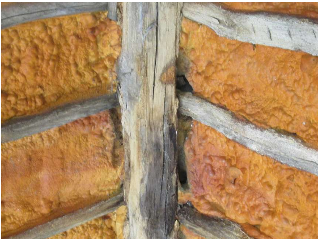
Photograph 8: Interior view of Building 1, with gaps above roofing beam visible.
