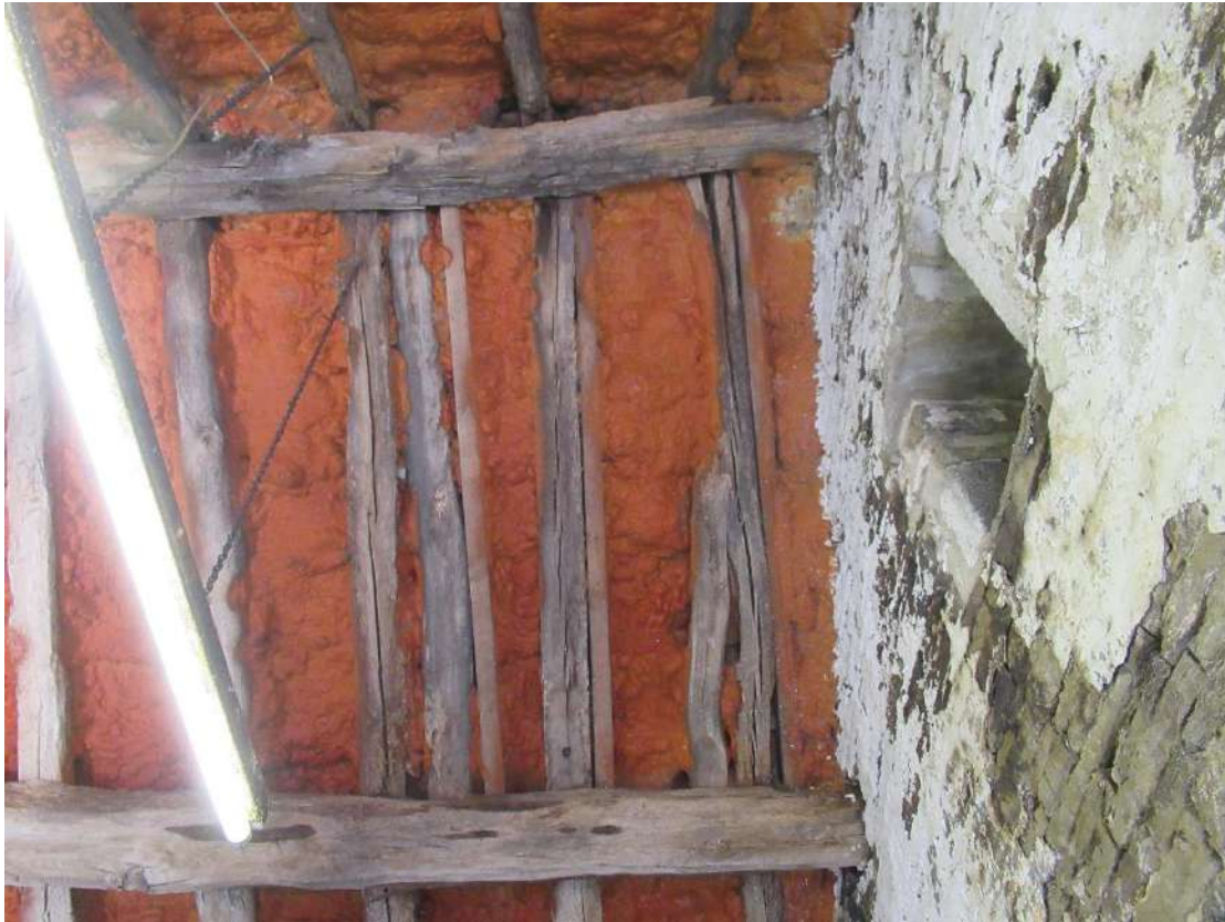
Photograph 7: Interior view of Building 1, with cracks in roofing beams visible.
