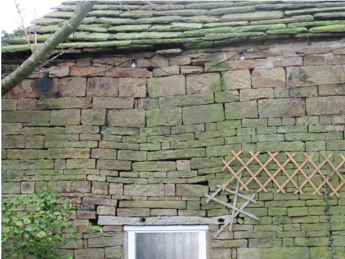
Photograph 5: Building 1 at the north-western elevation, with cavities in the wall visible between bricks.
