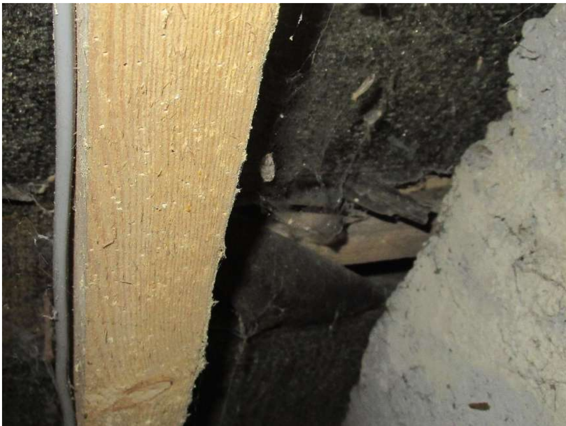
Photograph 14: Interior view of Building 2, with tear in bitumen lining.
