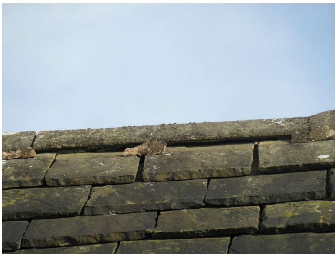
Photograph 12: Lifted ridge tiles on the south-western elevation of Building 2.
