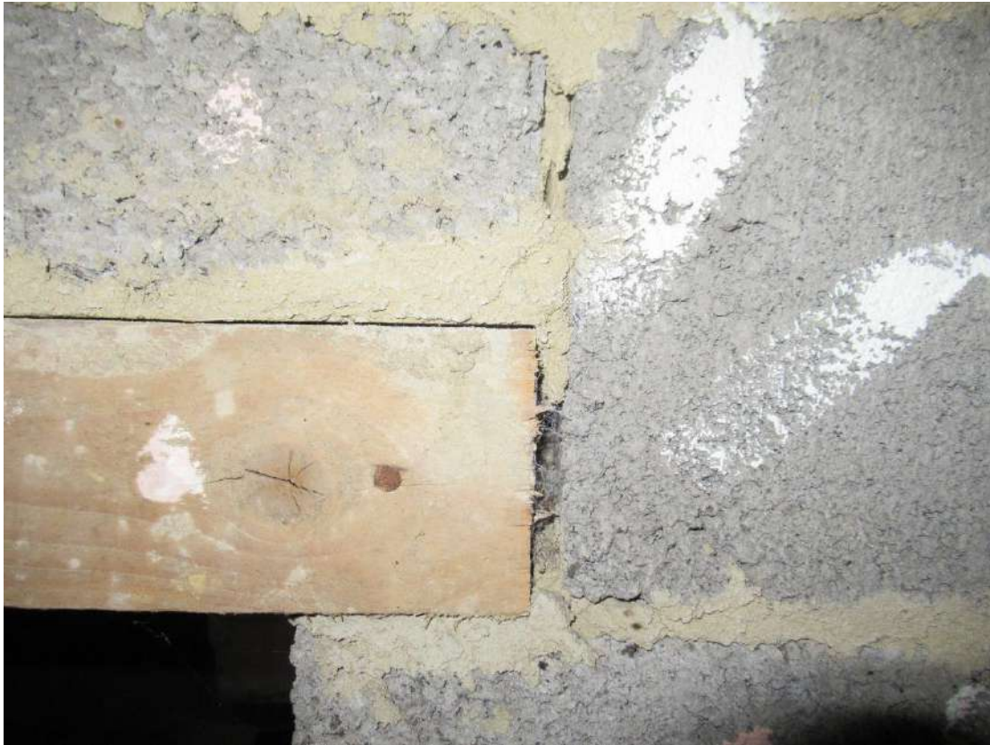
Photograph 13: Interior view of Building 2, with gap between the breezeblock and lintel.
