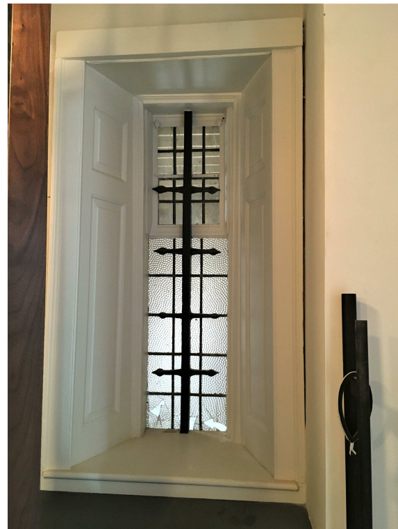
Window reveal and iron bar
