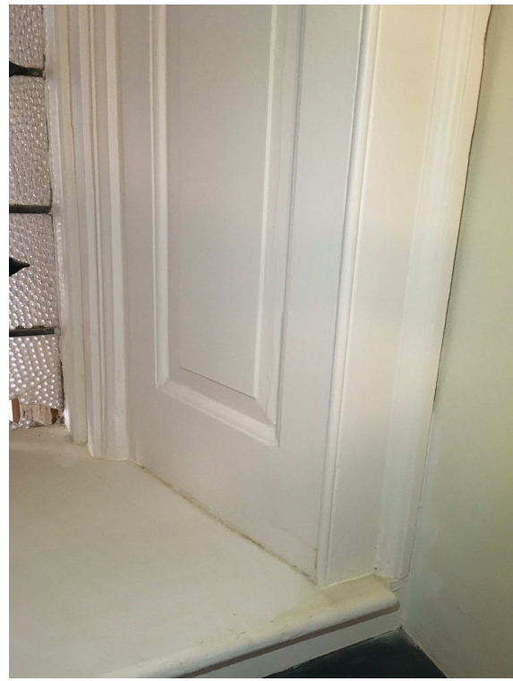
Timber panel reveal moulding and architrave
