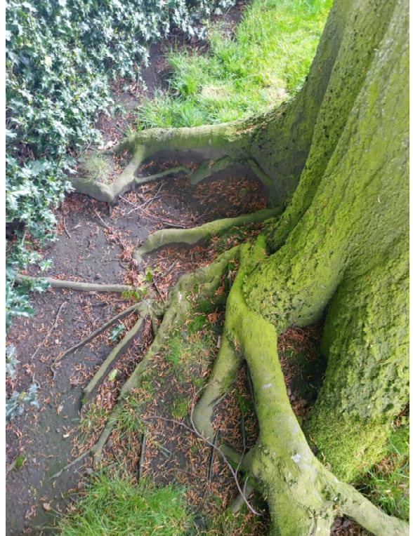
Photo 6: Exposed roots of T22.
