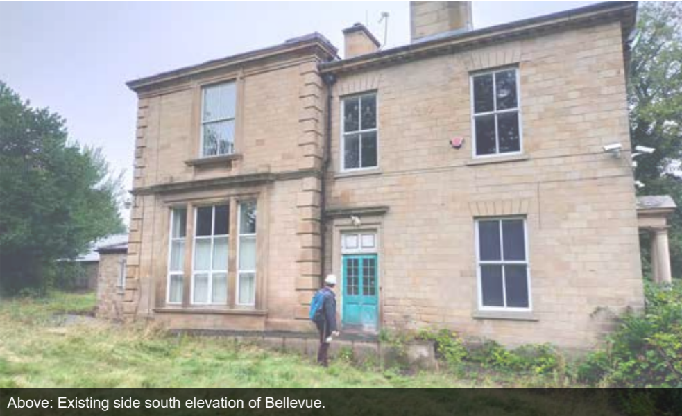
Above: Existing side south elevation of Bellevue.
