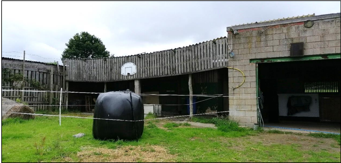
Plate 3. North end of B1 and adjoining B3
