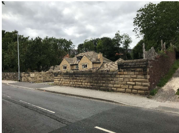
02. Site Frontage looking West
