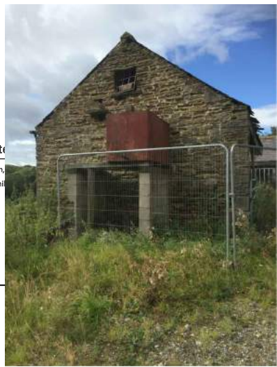
6. Facing west, above ground fuel tank on gable wall.
