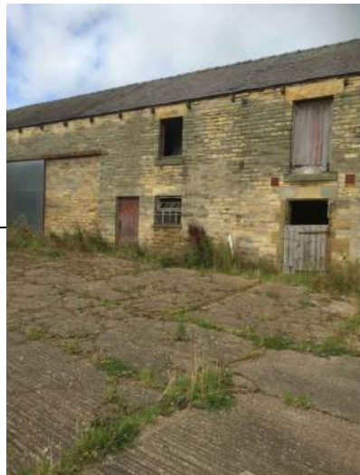
3. Facing northwest, view of the existing barn.
