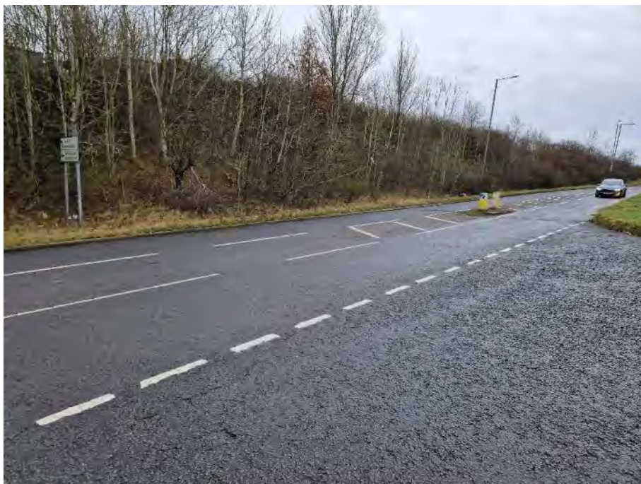
Photo 44 – View across junction with Ryecroft Bank
