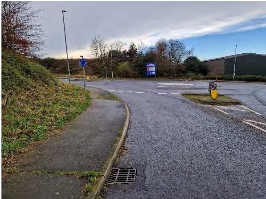
Photo 63 - View west of southern footway at mini roundabout.
