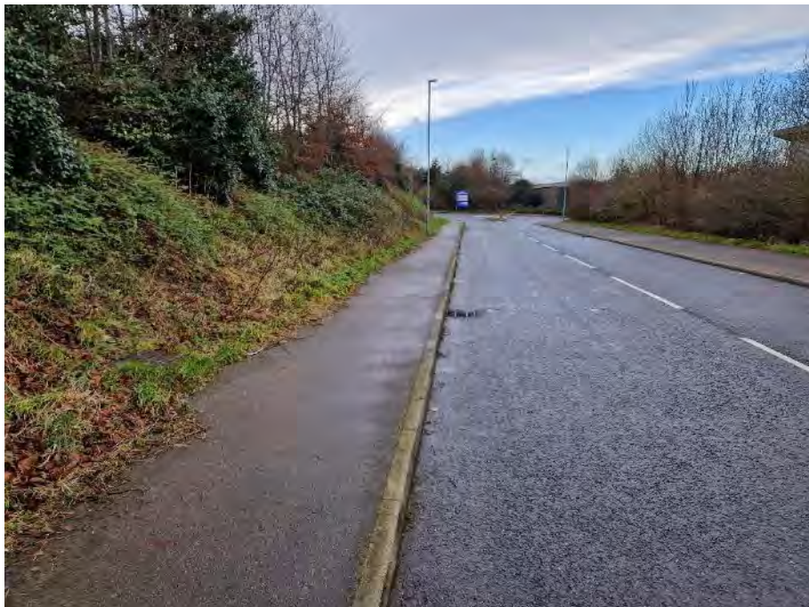
Photo 60 - View west of southern footway.
