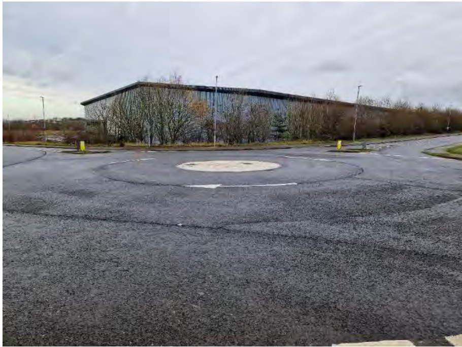
Photo 13 – View across roundabout.
