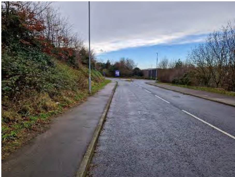
Photo 61 - View west of southern footway.
