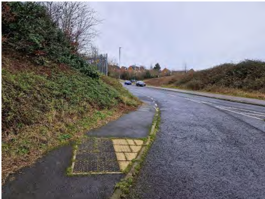
Photo 66 – Tactile paving on south eastern corner.
