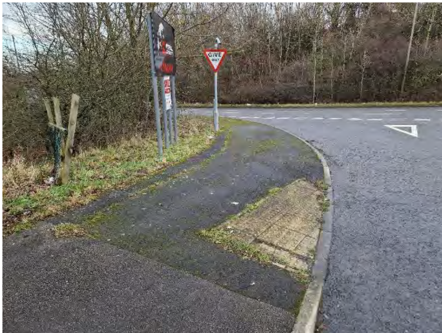
Photo 37 – Northern footway at Ryecroft Bank junction.
