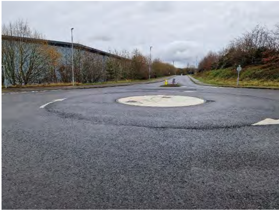
Photo 15 – View across roundabout
