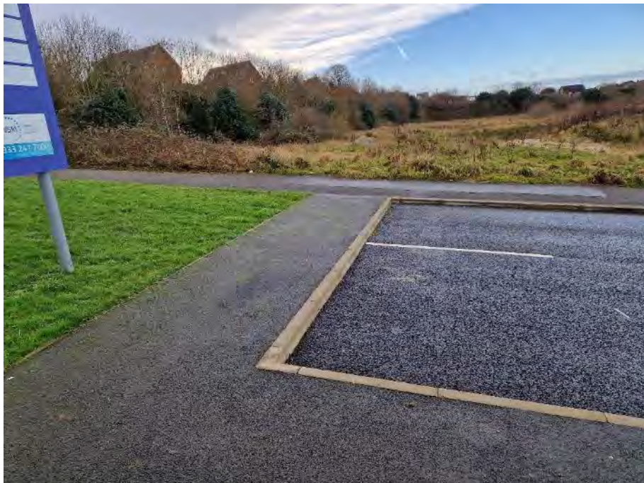
Photo 74 – End of carriageway.
