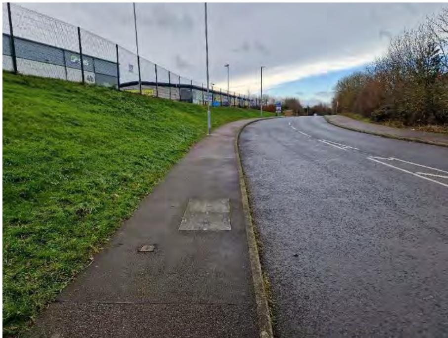
Photo 47 – View west of southern footway on Ashroyds Way.
