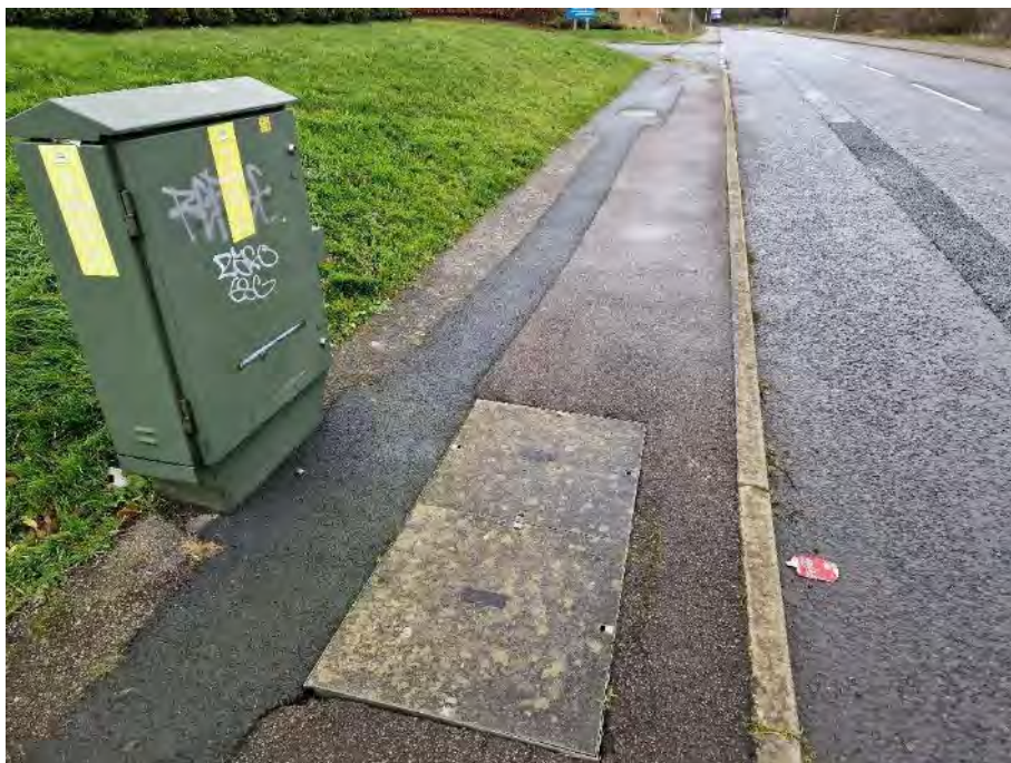
Photo 54 – BT chamber in front of Plot 4B.
