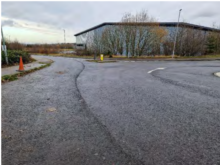
Photo 14 – View across roundabout
