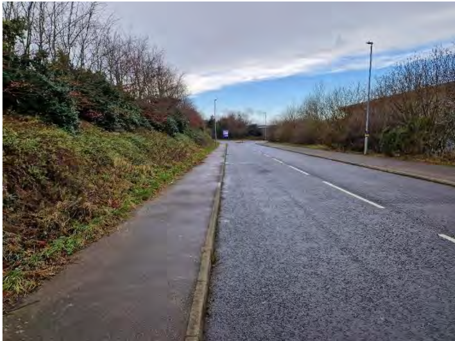
Photo 59 - View west of southern footway.
