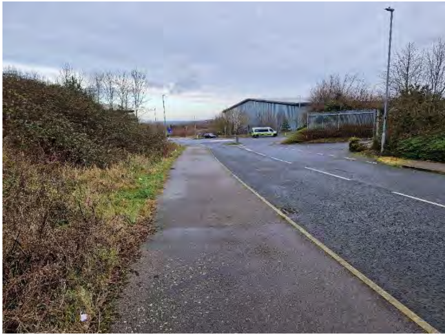
Photo 9 – View north on western footway.
