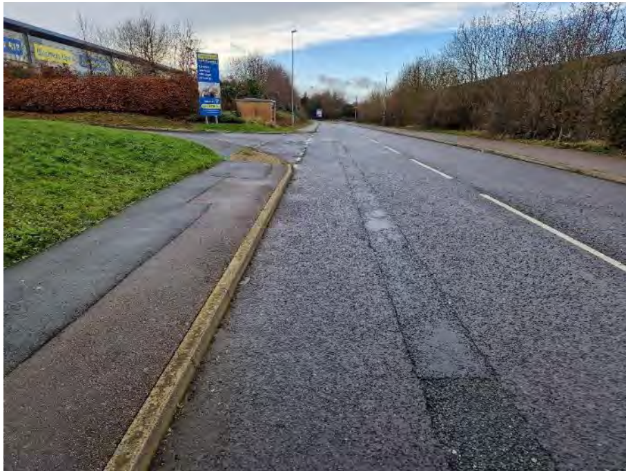
Photo 55 – Reinstatement in westbound lane in front of Plot 4B.
