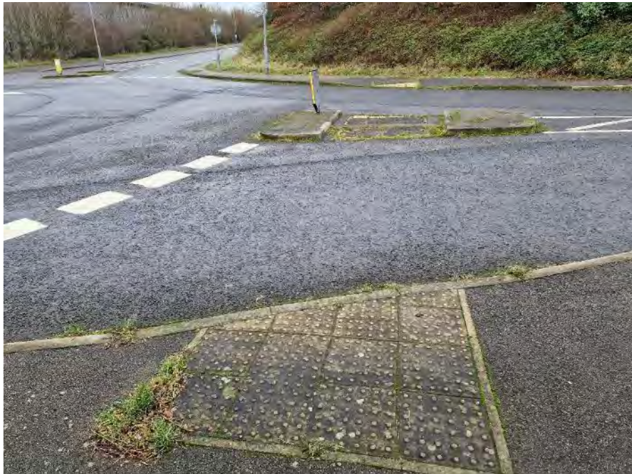
Photo 11 – View across tactile crossing on southern leg of roundabout.
