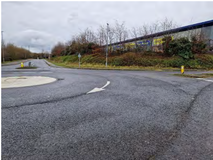
Photo 16 - View across roundabout
