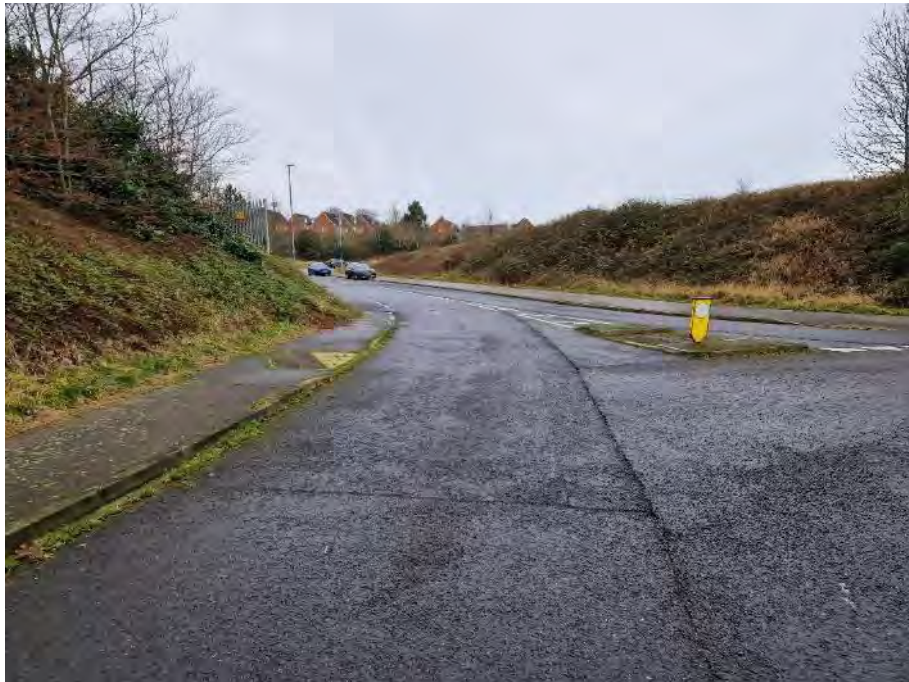
Photo 65 – View south from mini roundabout of eastern side of the road.
