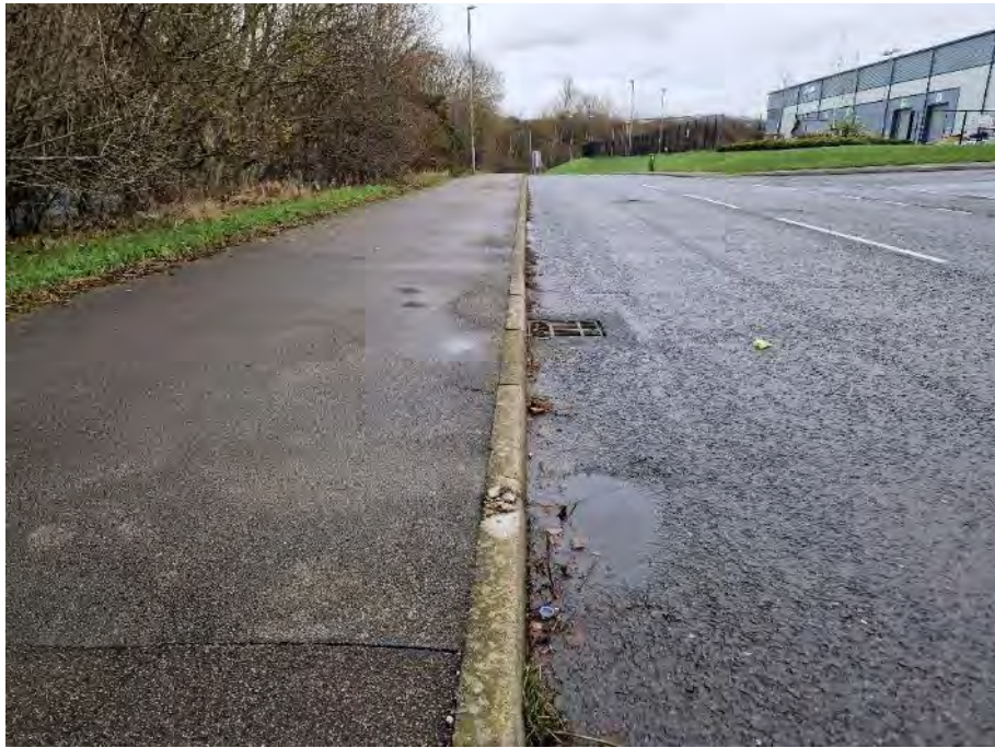
Photo 27 – Damaged kerb.
