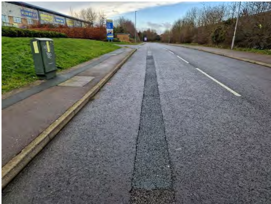
Photo 53 – Reinstatement in westbound lane in front of Plot 4B.
