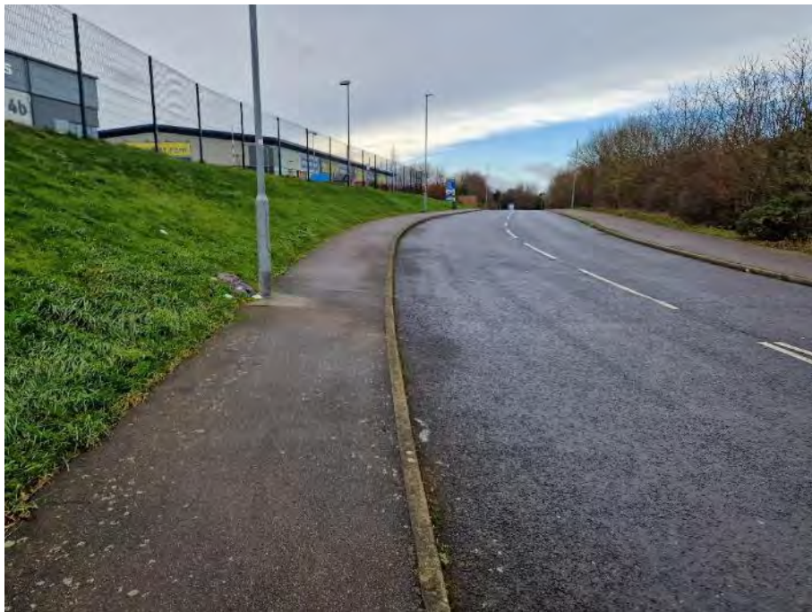
Photo 49 – View west of southern footway on Ashroyds Way.
