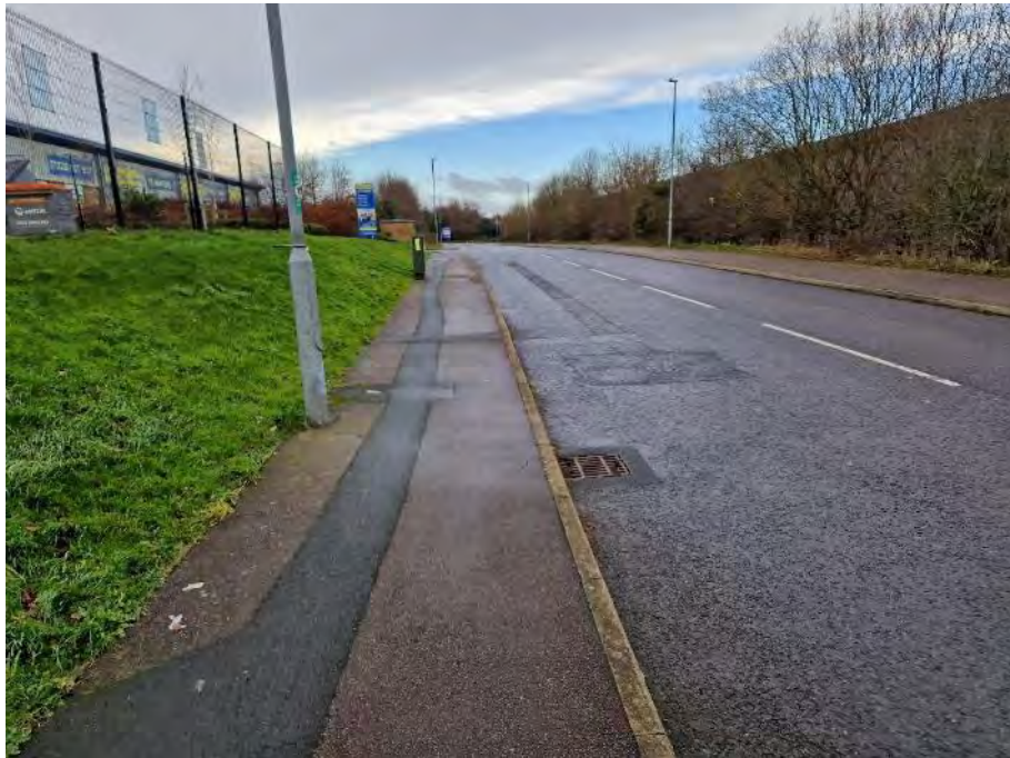
Photo 51 – View west of southern footway on Ashroyds Way.
