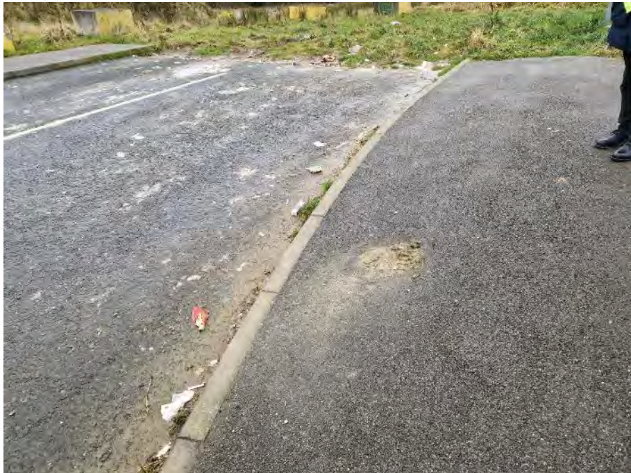
Photo 3 – Southern kerb line to Plot 3 entrance.
