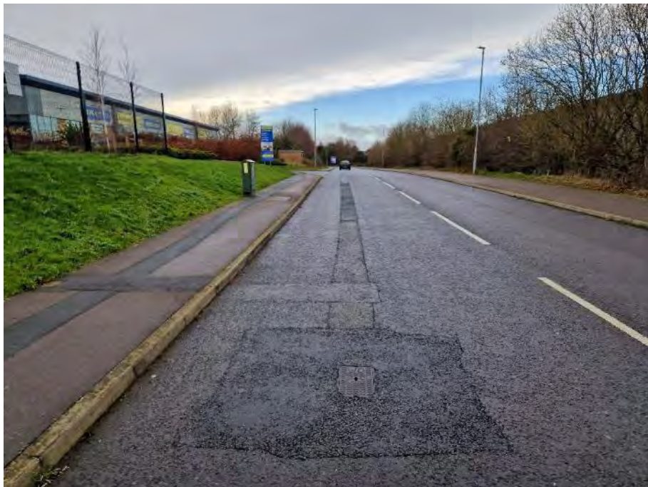
Photo 52 – Reinstatement in westbound lane in front of Plot 4B.
