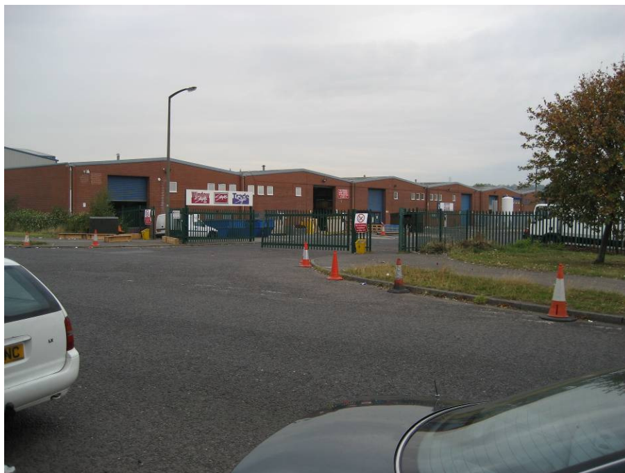
12a. Existing buildings, Nos 1-15 Valley Court providing glass toughening and office accommodation.
