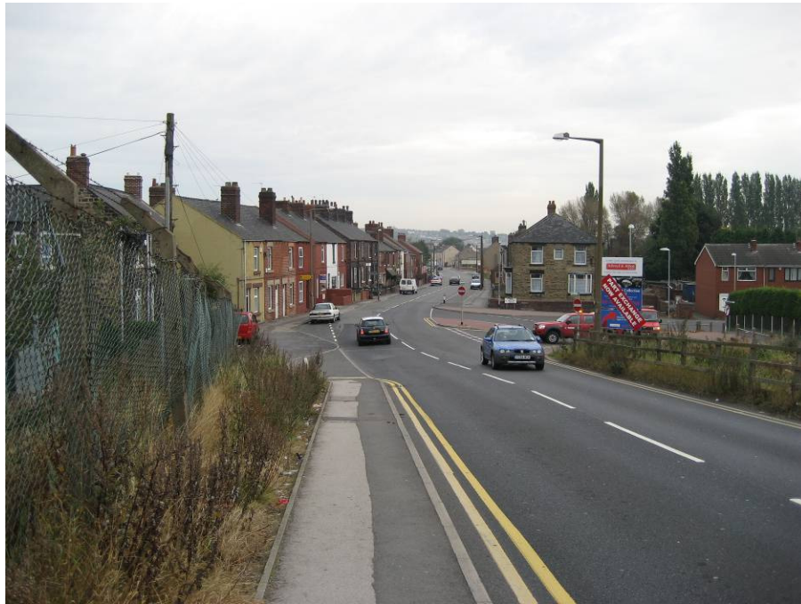
5. Approach to the site on Station Road from the A633 Wombwell by-pass illustrating existing terraced housing to the West of Valley Road.
