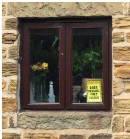
No jamb to poor stonework leaves a poor detail to seal from water penetration
