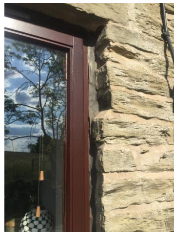
No jamb to poor stonework leaves a poor detail to seal from water penetration
