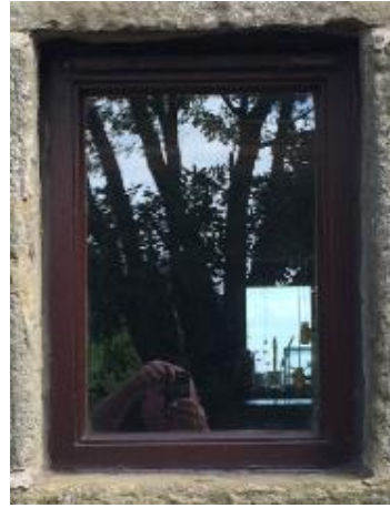
Small Lounge Window to Westerly Elevation
