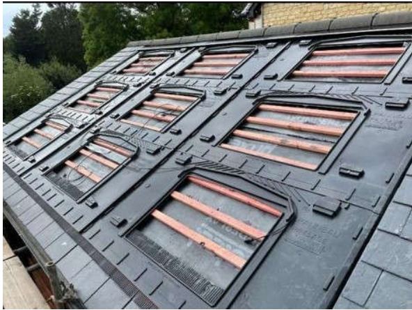
Fig 01. Panels installed in similar blue slate roof.
