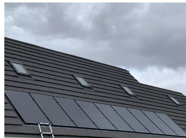
Fig 03. Completed panel installation (not blue slates).
