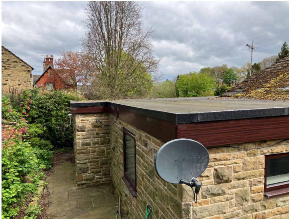
Fig 06. Flat roof extension to rear and typical random stone walling.
