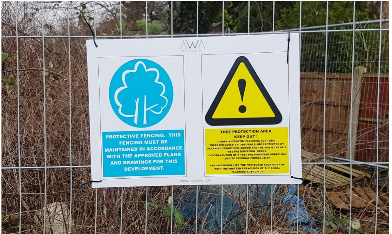
Figure 6: Example of A3 correx tree protection warning sign fixed to fencing panel
