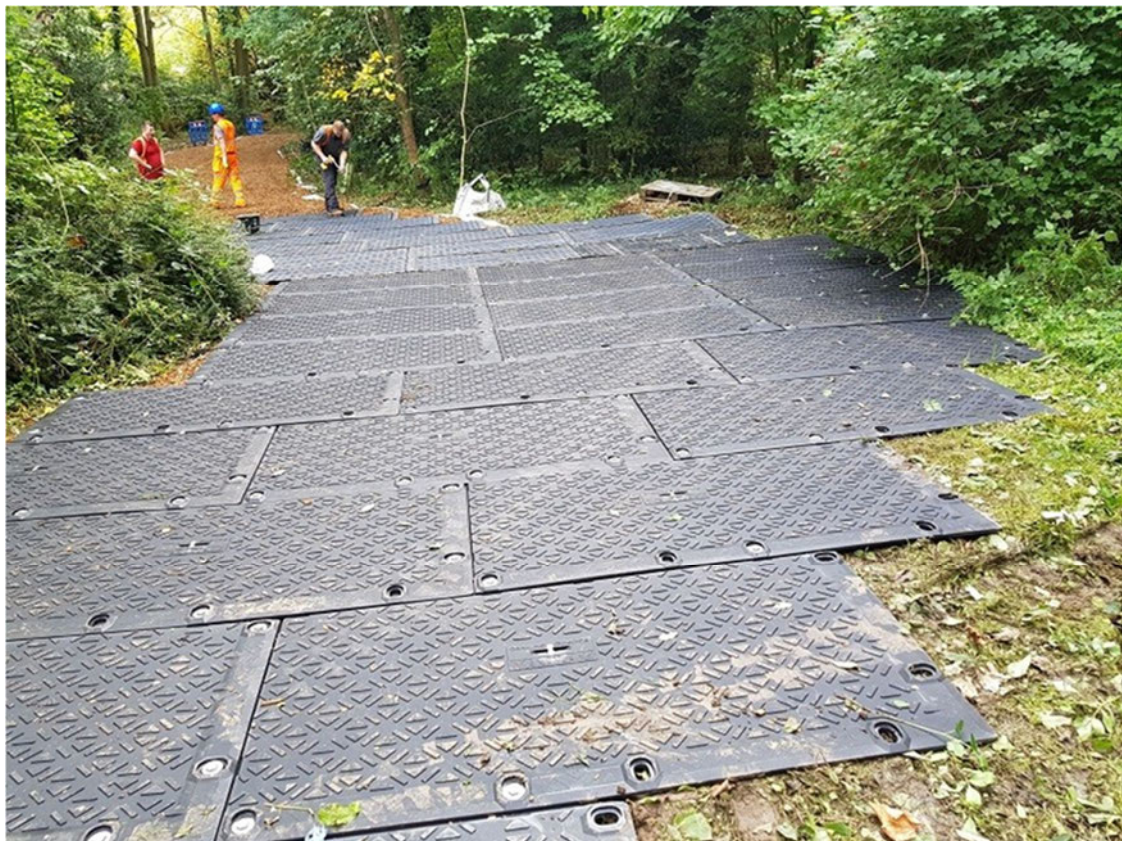
Figure 7: Interlinked ground protection boards placed on top woodchip
