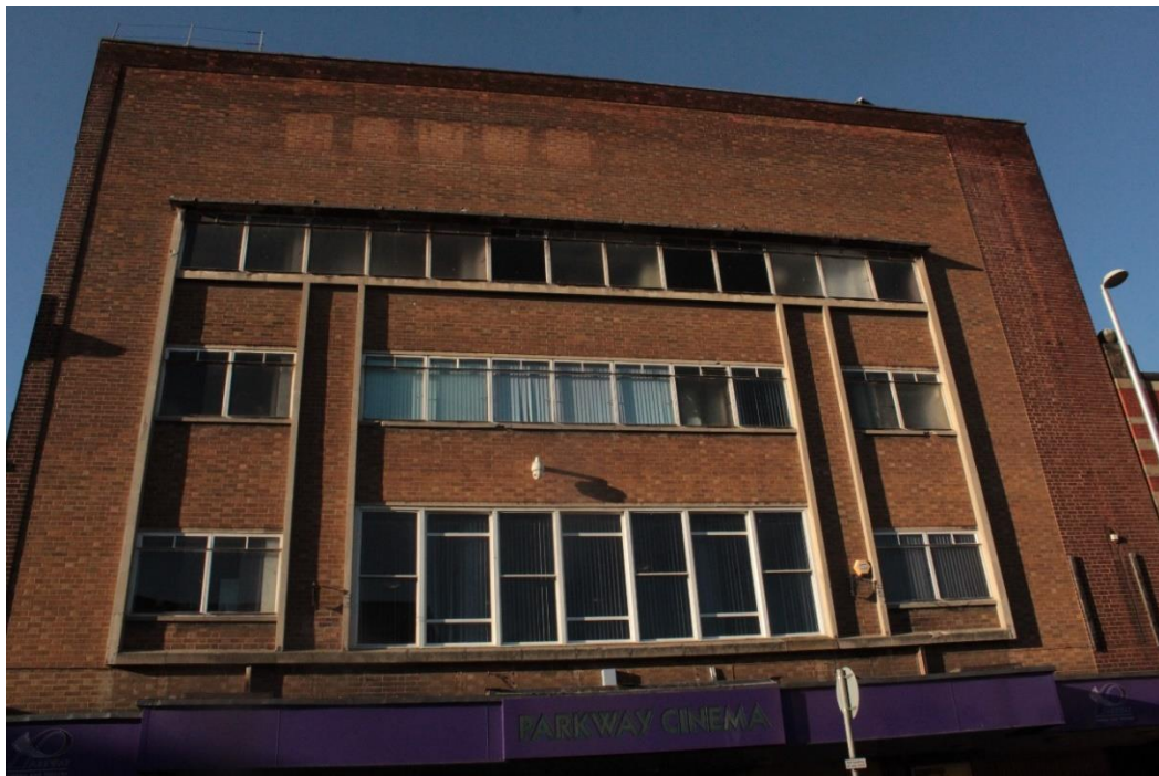
Fig 02. The brick and concrete inset panel on the Eldon Street elevation.
