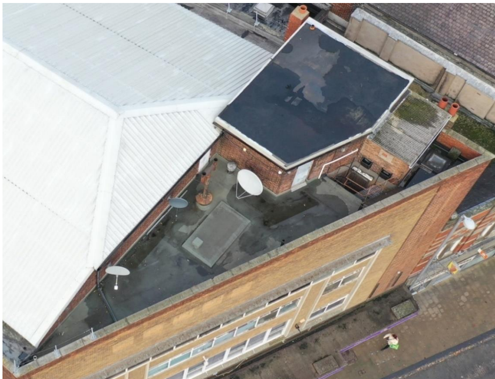
Fig 17. The triangular area of flat roof finished with green bitumen-based roofing felt
