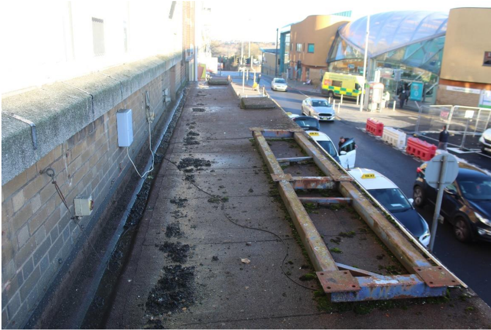
Fig 29. The steel frame on the canopy above the main entrance.
