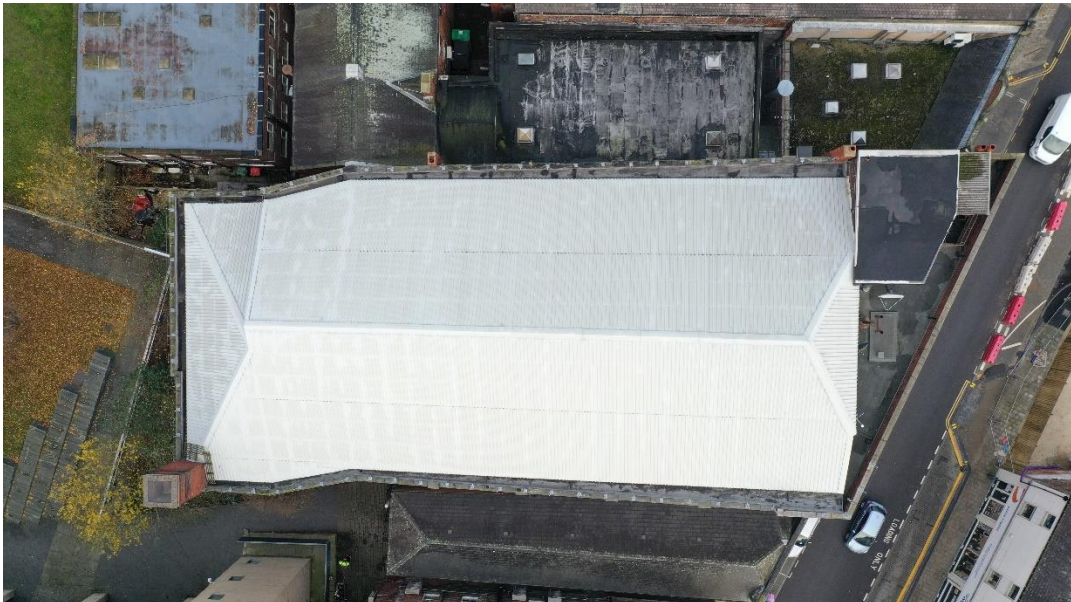
Fig 04. The roof of the cinema (taken by drone from above).
