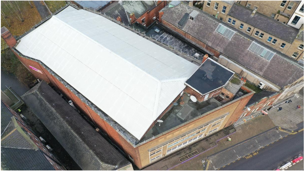
Fig 03. The roof of the cinema (taken by drone from the south-east).
